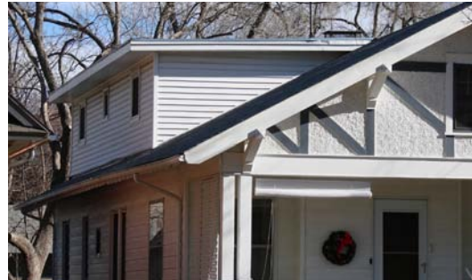
Inappropriate dormer scale
