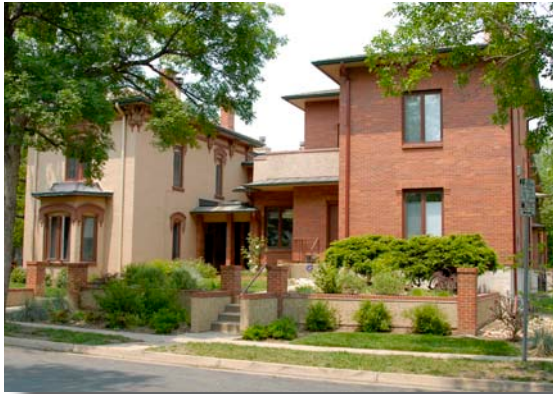
Appropriate scale, massing and materials of addition, plus simplified but complementary detailing
