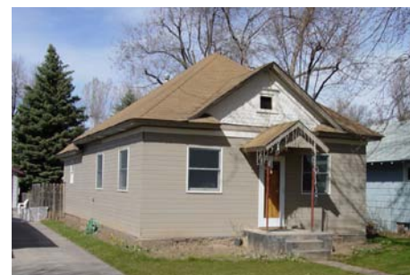
Inappropriate window replacement, where window openings have been reduced in size.
