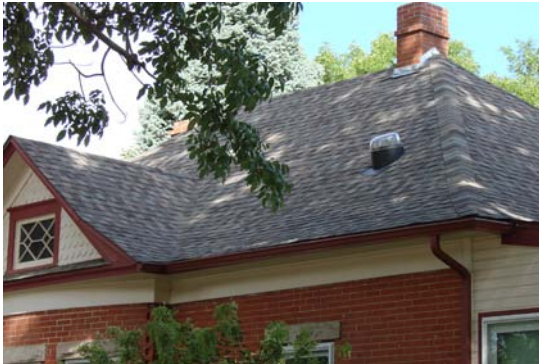
Appropriate solar "tube" installation
