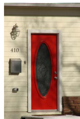
Inappropriate replacement door
