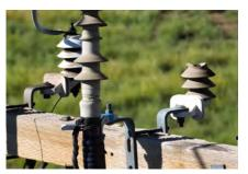
These photos show examples of proactive maintenance that helps prevent outages before they happen. From left to right: evidence of electrical arcing, infrared images of an overheating fuse and damaged lightning arresters.
