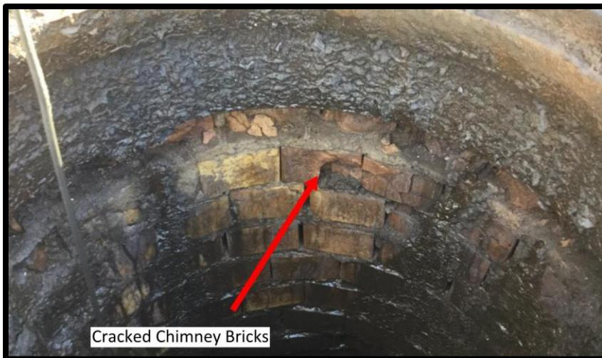
*Figure 13 – Cracked Chimney Bricks in Stormwater Manhole*
