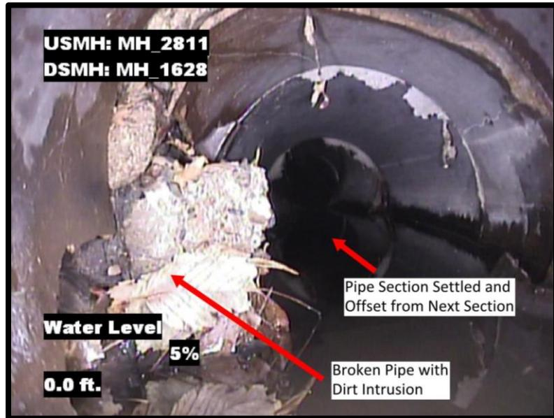
Figure 10 – Structurally Deficient Stormwater Pipe at Sixth & Cleveland
