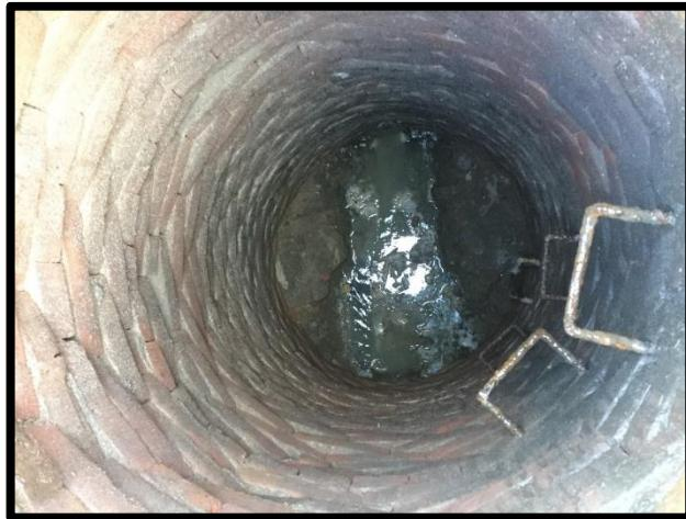
*Figure 8 - Existing Brick Sanitary Sewer Manhole 3420*
