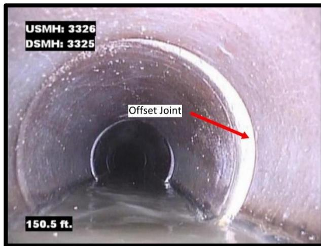
Figure 5- Offset Joint in 10-inch Sanitary Sewer Under Garfield Avenue
