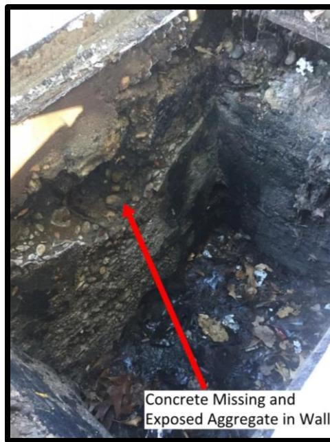
*Figure 12 – Wall Damage at Inlet by Fourth & Railroad*
