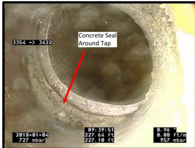
Figure 7 - Offset Sewer Tap Connection Sealed with Concrete
