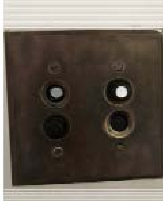
Many of the rooms still have push-button switches even though the patent for the toggle-light switch patent was obtained in 1916.
