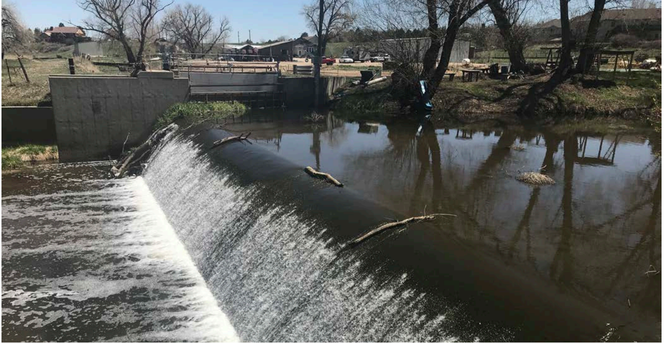
Hillsborough Ditch diversion structure
