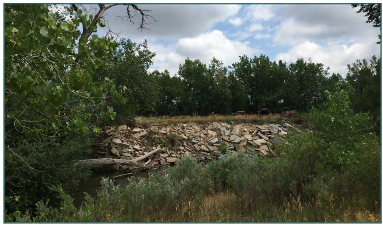
Exposed concrete and debris creates an unsightly and potentially hazardous riverbank condition that should be removed prior to construction.
