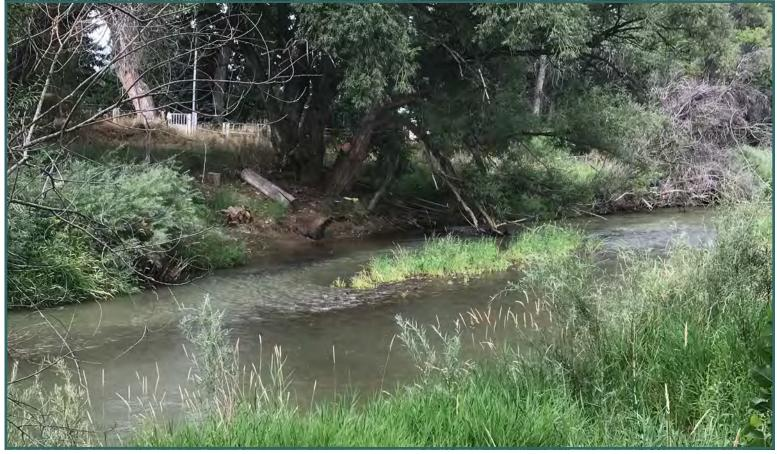
In some areas where sediment deposits from the flood persist in the river, vegetation is becoming established. As vegetation becomes established, the roots further stabilize and anchor deposited sediments leading to continued aggradation This is especially problematic at bridge crossings of the river where sediment accumulation reduces bridge and culvert capacity.
