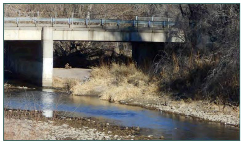
Bridge and channel maintenance to clean out accumulated sediment and vegetation is one of the most cost effective ways to increase conveyance capacity. This will not eliminate the need for additional bridge and culvert capacity and some crossings; however, given constraints on funding, maintenance is a cost effective way to make incremental improvements and reduce municipal liability in a future large flood event.
