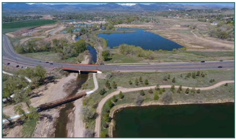
The pedestrian bridge across the Big Thompson River upstream, of Wilson Avenue was replaced following the 2013 flood as a part of the Wilson to Taft Flood Recovery Project. This project for restoration of approximately 4,400 feet of the river included trail reconstruction, repair of erosion, and creation of floodplain benches in addition to the bridge replacement. This work was partially funded by FEMA grants in combination with City contributions.
