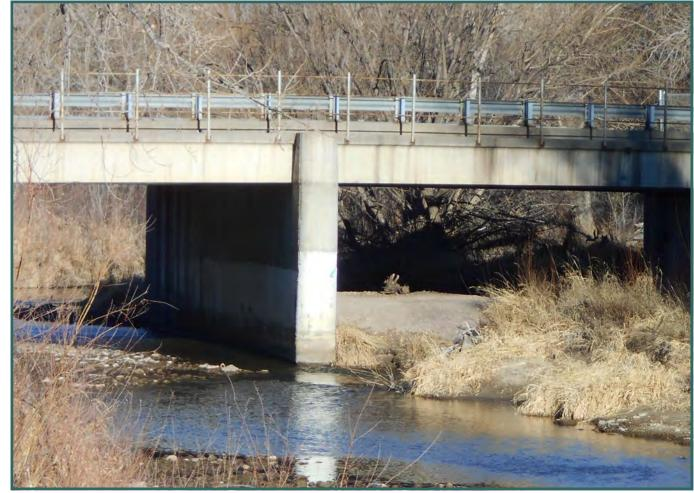
Some portions of the river corridor have a natural character and require little maintenance; however, in other areas, a better maintenance program is needed. As an example, cleaning sediment and vegetation from the northern cell of the Taft Avenue Bridge would increase conveyance capacity significantly.
