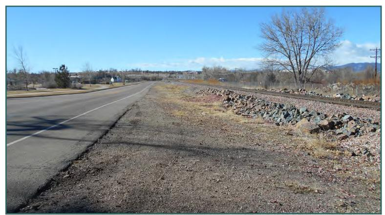
View along Railroad Avenue looking south from bridge. This photo illustrates the elevation difference between the railroad and the road to the east. The railroad acts like a dam, backing up floodwaters due to existing bridge and culvert conveyance limitations. Fairgrounds Park lies immediately east of the road, and in 2013, flows overtopping the railroad and flowing through ballast material caused significant damages in the park.
