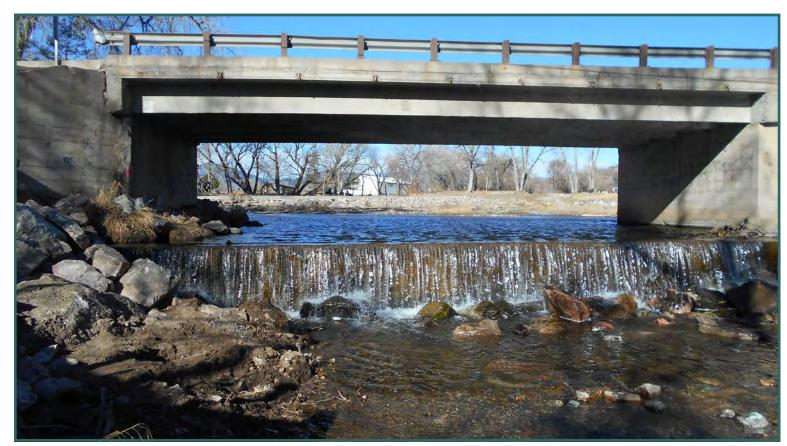
Vertical drop on downstream side of Namaqua Avenue Bridge. While this drop dissipates energy and aids in grade control, under some flow conditions, the drop creates dangerous hydraulic currents. At least one drowning death is known to have occurred at this location. This drop will be removed and replaced with a more gradual drop as a part of the Larimer County bridge replacement project, which will improve public safety in this location.
