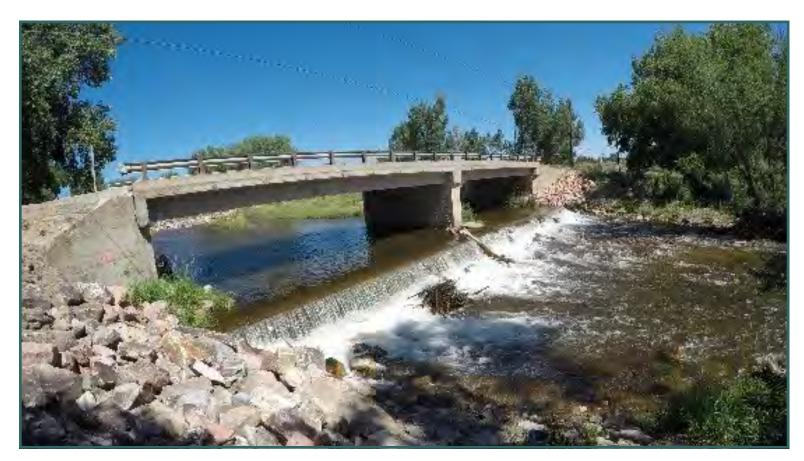
This low head dam at Namaqua Avenue is one of two fish barriers over a short distance of the river. The Rist-Goss diversion dam is another, just upstream of Namaqua Avenue. Larimer County has plans to replace the low head dam shown with a new drop that will allow for fish passage, and BTWC is evaluating options for the Rist-Goss diversion dam.
