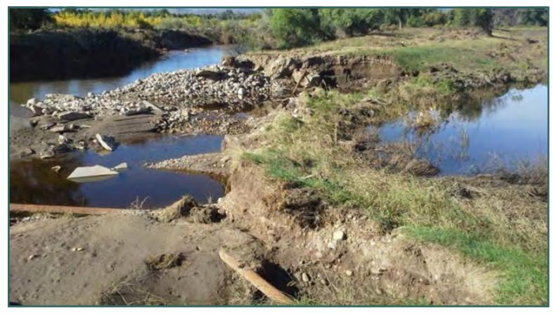
Return point of south overbank and avulsed flow from gravel pits to the main river channel approximately 400 feet upstream from Wilson Avenue. The main channel of the river is shown on the left and the gravel pit is on the right. An exposed utility line can be seen in the foreground. Providing armored spillways meeting the criteria in Appendix D are recommended to avoid these types of damages in future large flood.
