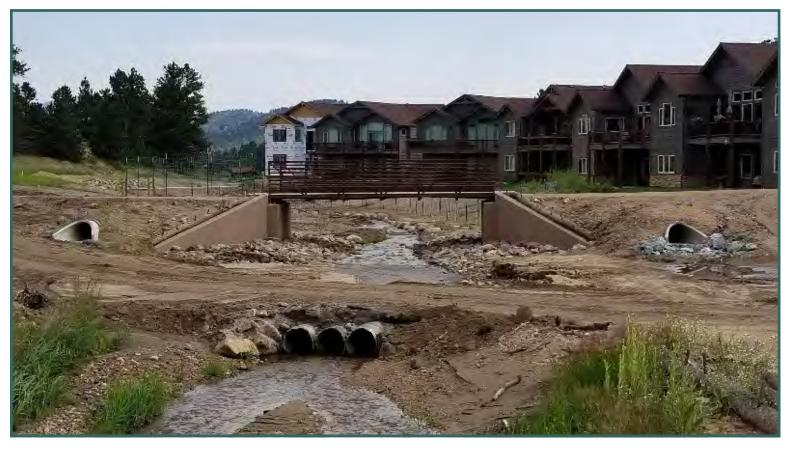
Floodplain relief culverts are a good way to provide excess capacity at road crossings for infrequent events, especially in a wide floodplain like the Big Thompson's where flows spread out hundreds of feet in some locations and develop split flow paths through gravel pits.
