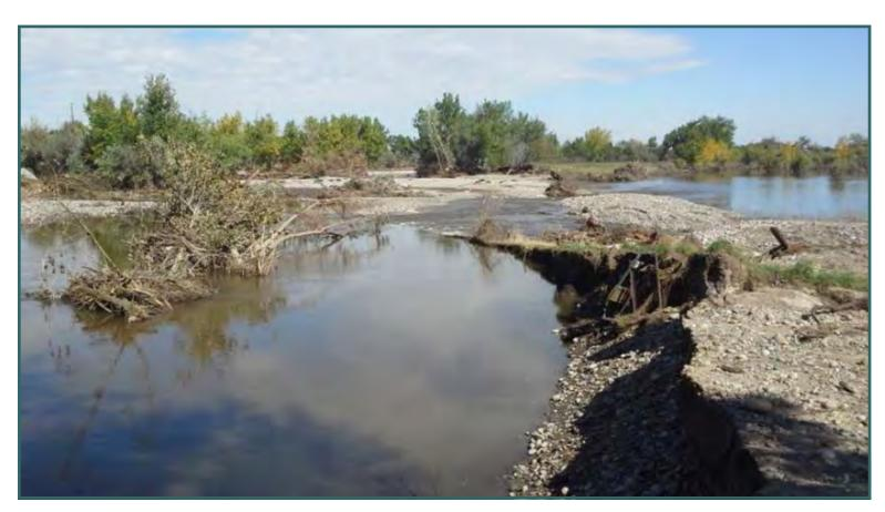
Avulsion into gravel pits just downstream of wastewater treatment plant outfall channel. Gravel pits stored significant quantities of runoff during the September 2013 flood; however, due to the extreme amount of total precipitation, runoff volume, and the uncontrolled nature of flows between the river and the gravel pits and return flows, the effects of this storage were diminished in the 2013 flood.
