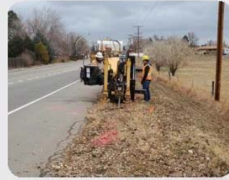
Start of Boring and Conduit Installation
