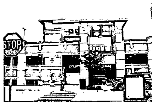
Figure 16-15b – Cross Street Parking Garage Example
