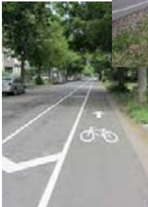
Improved bicycle lanes with street trees
