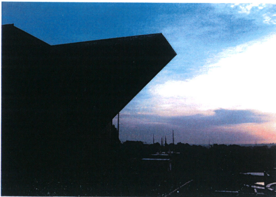
#3 - Headworks odor control exhaust
