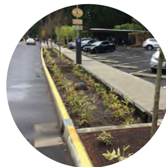
Curb cuts help capture and beneficially use stormwater runoff from the streets and sidewalks.
