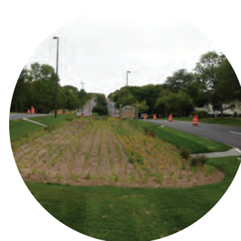
Bioswales work by slowing and filtering stormwater, especially from large, impervious areas, like parking lots or roadways.
