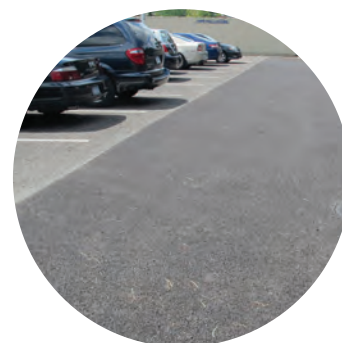
Pervious pavement reduces hardscapes, providing more opportunities for groundwater infiltration to lessen stormwater runoff.
