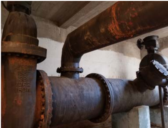
Left: Existing 36" Gate Valves to be Replaced Below: Existing Mod Valve
