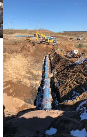
Left: New 30" Morning Drive Water Main Connecting to existing piping at 29 th Street tank.
