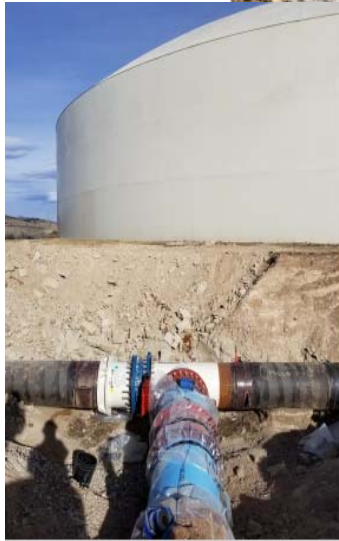
Left: New 30" Morning Drive Water Main Connecting to existing piping at 29 th Street tank.
