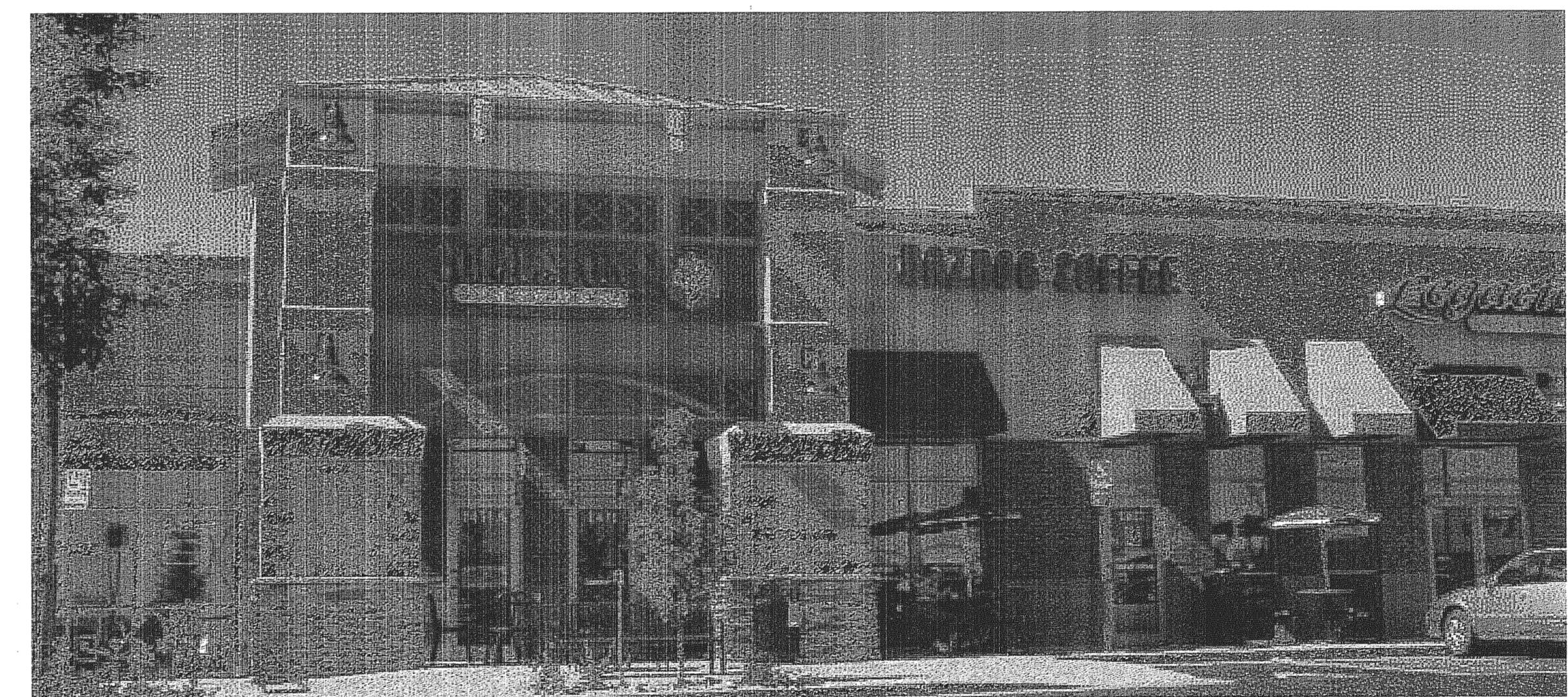
EXAMPLE: HIGH QUALITY EXTERIOR BUILDING MATERIALS INCLUDING SMOOTH FACE CONCRETE BLOCK USED TO PROVIDE VARIATION IN COMBINATION WITH OTHER TEXTURED MATERIALS.
