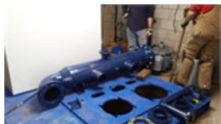
The Mariana Butte pumpstation was installed in 1991 and the fire suppression was added in 2009. The controller will be updated to a variable frequency drive and the steel piping, pumps, and motors will be replaced to allow for improved energy efficiency and enhanced operation. Due to the update of the variable frequency drive, the pump station replacement should qualify for the Platte River Power Authority Efficiency Program.
