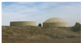
The 29th Street steel tank is one of the most utilized storage facilities supporting over a quarter of the City's water customers. This project will provide a second 5.0 million gallon (MG) storage tank at this critical location.
