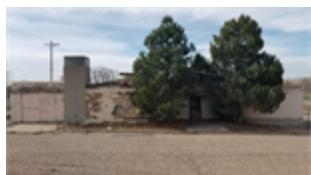
The City has an abandoned wastewater treatment plant located at Railroad Ave. and 3rd St. SE. There is an existing active 15" sanitary sewer that runs through the abandoned plant and poses a safety concern. This project will re-route the sanitary sewer out and around the abandoned plant site.
