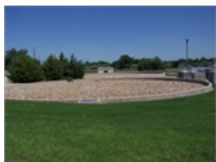
This project is for the demolition of the existing trickling filter basins and construction of a third primary clarifier to increase capacity of the primary treatment system to 12 MGD. The primary clarifier will be constructed in the area now occupied by the decommissioned trickling filters.
