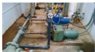
Currently there is a pump station that feeds the upper loop of homes in the Namaqua Hills Subdivision. The pump station was built in 1962 and the components have reached the end of their useful life. The pumps, piping, and SCADA equipment is to be replaced to ensure reliable service to customers.
