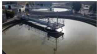
In an effort to reduce odors from the WWTP the Department will cover the primary clarifiers and other associated odor causing processes. As a result of covering the clarifiers some equipment and surface coatings will have to be replaced or rehabilitated to combat resulting sewer gases.
