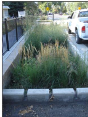
An annual program to retrofit stormwater quality treatment measures into existing stormwater systems in order to improve the quality of waters receiving stormwater runoff. The program includes an annual expenditure of \$75,000 - \$100,000 for retrofit projects as it has historically along with funding for the 1% for the Arts.
