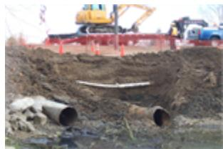
This project will line the existing culvert and install a second one under 29th Street at the outlet to the Benson Park pond. The existing culvert is corrugated metal and is in the process of failing because of significant corrosion. The purpose of this project is to repair the crossing before the existing culvert collapses.
