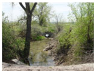
This project will mitigate existing erosion problems within the Boyd Lake Outlet Ditch between Eisenhower Boulevard and 5th Street, directly east of Kohl's. We jointly utilize this irrigation return flow ditch to convey stormwater runoff to the Big Thompson River. In accordance with the 1984 agreement between the City and the Greeley & Loveland Irrigation Company, we are required to make necessary improvements to the ditch in order to convey stormwater to the river.
