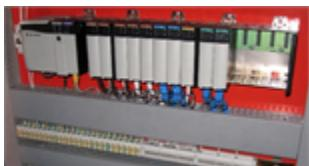
Replace 7 Allen Bradley SLC 500 PLCs with new Allen Bradley Controllogix PLC controllers. Project includes programming and integration for transition from RSLogix 500 to RSLogix 5000 and replacement of existing SLC level I/O.
