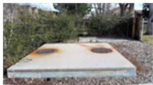
The Eastside sanitary sewer lift station has two forcemains which discharge into a vault before flowing via gravity through the collection system. The vault's condition is worsening due to H2S gas (from sewer gases) and will need repaired and/or replaced.
