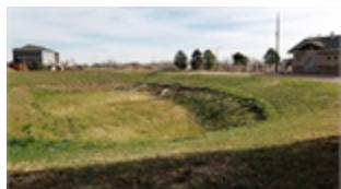
The Eastside Lift Station has an overflow pond situated next to it should there ever be a backup of sanitary sewer flows. It is the City's desire to convert this pond into a concrete vault to serve the same purpose. The vault would allow for better cleaning and less environmental impact in the event of an overflow discharge.
