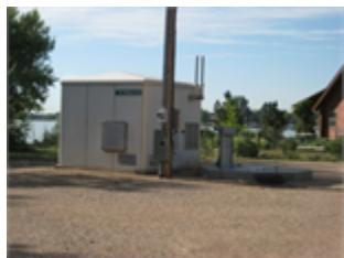
This is an aging lift station located near Horseshoe Lake. Proposed improvements are not exactly known at this time, but will likely include: emergency overflow storage, lining of existing wetwell, and replacement of piping, valves, and controls.
