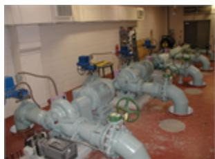
The existing pump station situated at 29th St. and Cascade serves the P1 pressure zone. Currently there are two 50-hp and two 100-hp pumps in the pump station. Due to increased demand within the pressure zone the two 50-hp pumps are to be replaced with 100-hp pumps. This will ensure that current and future customers receive sufficient water pressure and supply.
