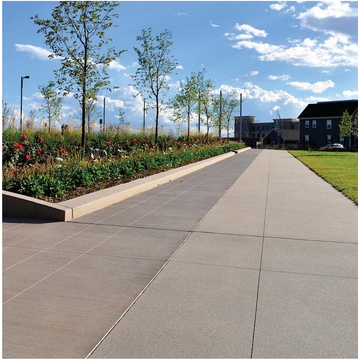
Concrete Grey concrete with saw cut joints
