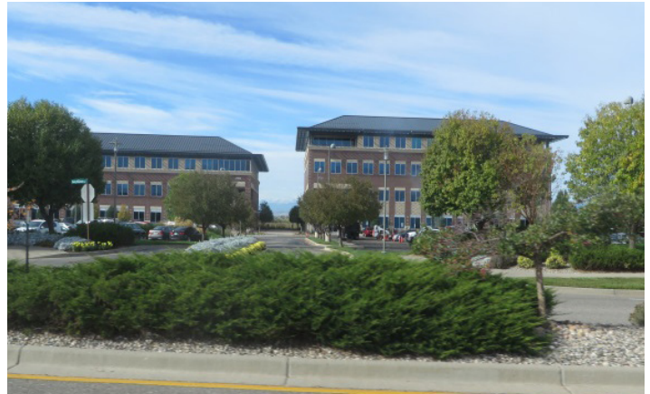
Office park on Rocky Mountain Ave.
