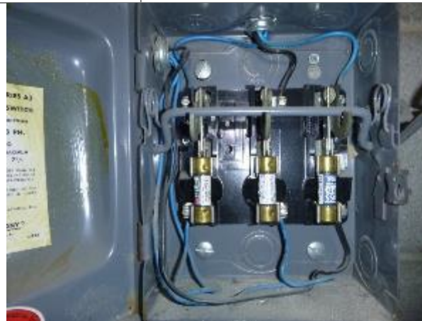
Photo #76 HA-74, Mechanical Room, assumed fuses
