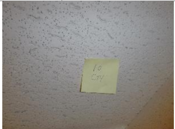
Photo #16 HA-10, 2' x 4' tan ceiling tile with thick horiz. fissures and holes
