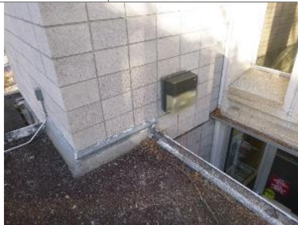
Photo #96 South exterior, suspect mercury-containing high intensity discharge lamp
