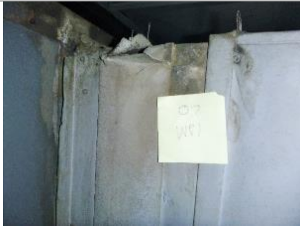
Photo #13 HA-07, bray vibration joint cloth
