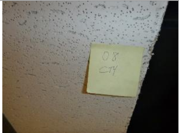
Photo #14 HA-08, 2' x 4' lt gray ceiling tile with horiz. fissures and pinholes
