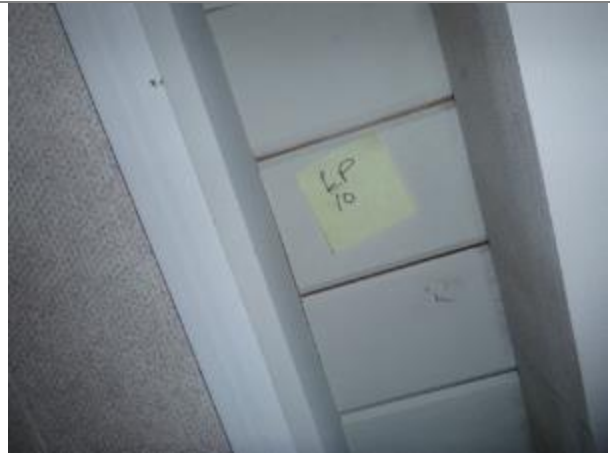
Photo #80 LP-10, wood ceiling deck with light gray paint
