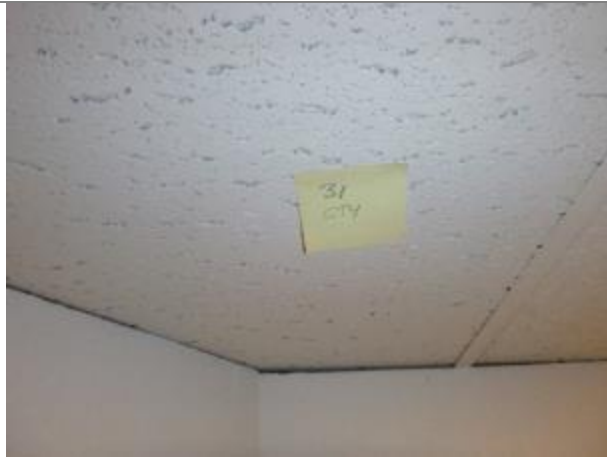
Photo #37 HA-31, 2' x 4' pink ceiling tile with horizontal fissures and wide spaced holes
