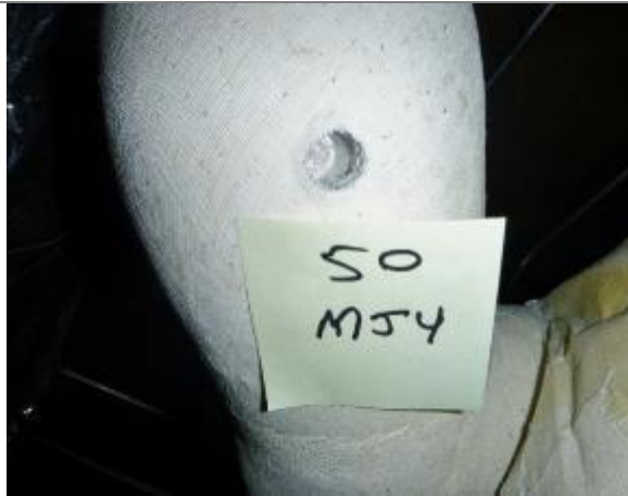
Photo #55 HA-50, white roof drain pipe fitting insulation
