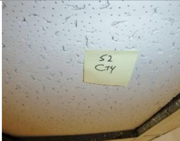
Photo #57 HA-52, 2' x 4' white ceiling tile with chicken feet fissures and pinholes
