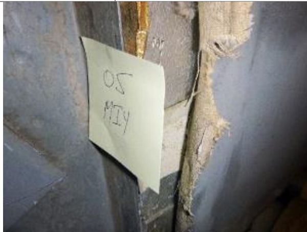
Photo #11 HA-05, gray tape with gray canvass wrap duct insulation
