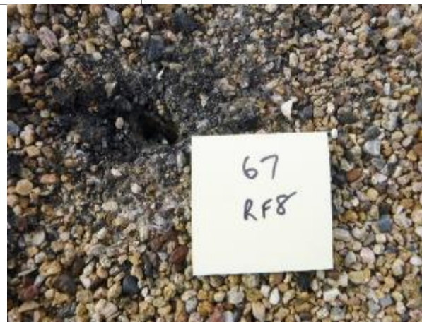
Photo #72 HA-67, brown built-up asphaltic roofing with brown insulation and styrofoam
