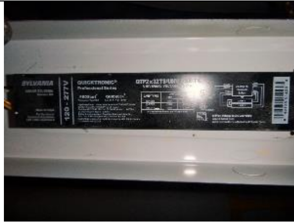
Photo #92 Mechanical Room, non-PCBs ballast
