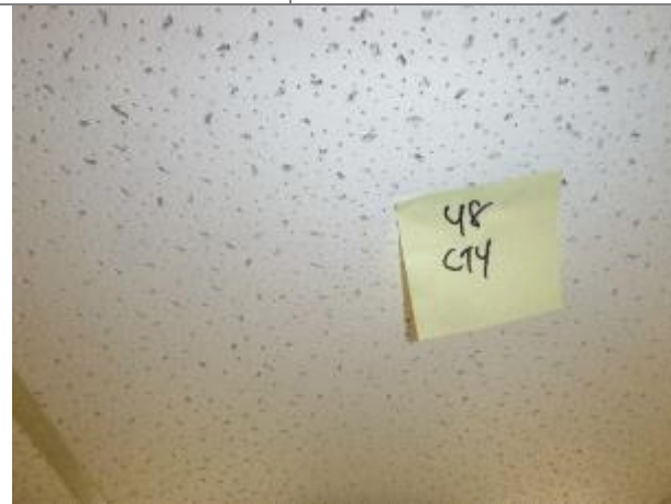
Photo #53 HA-48, 2' x 4' tan ceiling tile with small pinholes and large star pinholes
