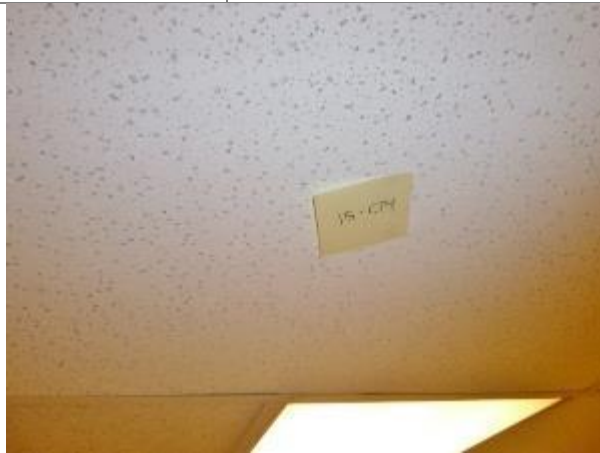
Photo #21 HA-15, 2' x 4' lt gray ceiling tile with small and medium holes
