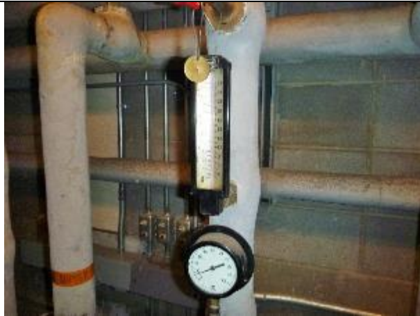
Photo #97 Mechanical Room, suspect mercury-containing thermometer
