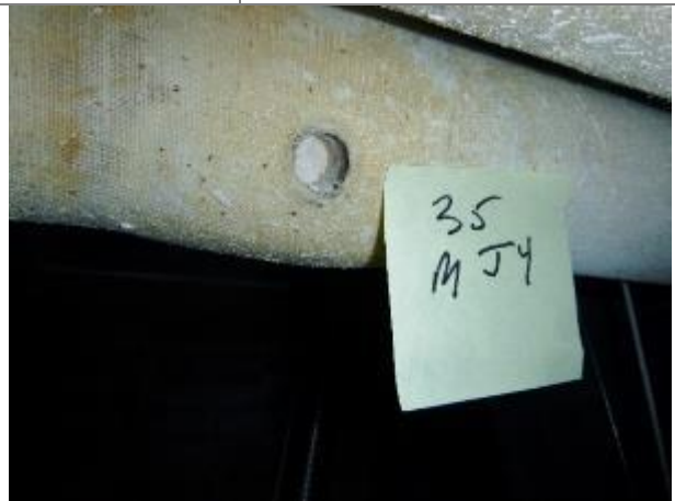
Photo #40 HA-35, white hot and cold water pipe mudded joint fitting
