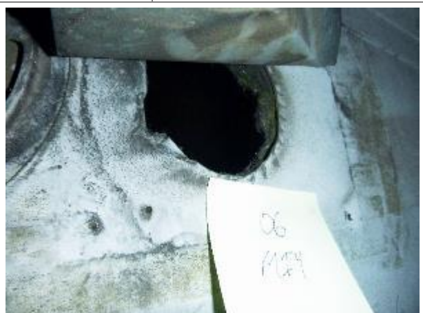
Photo #12 HA-06, black coating on tan fiberglass, duct insulation
