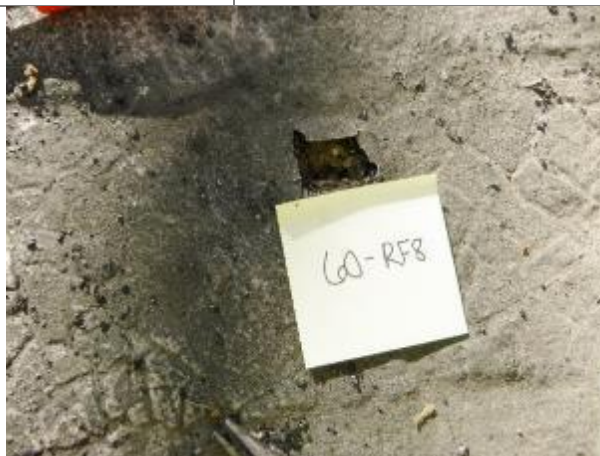
Photo #65 HA-60, white and black built-up roofing with tan insulation
