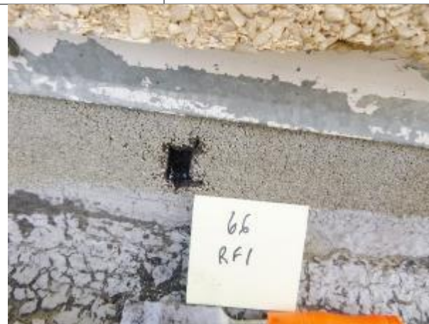
Photo #71 HA-66, gray rolled-on flashing with black tar and silver paint
