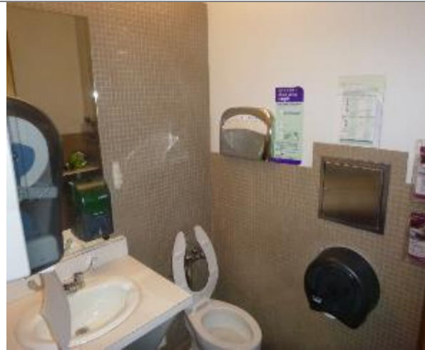
Photo #74 HAs-71 & 73, Health Dept. bathrooms, assumed ceramic tile and mirror mastic
