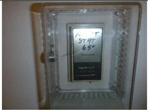
Photo #98 Conference Rooms, suspect mercury-containing thermostat
