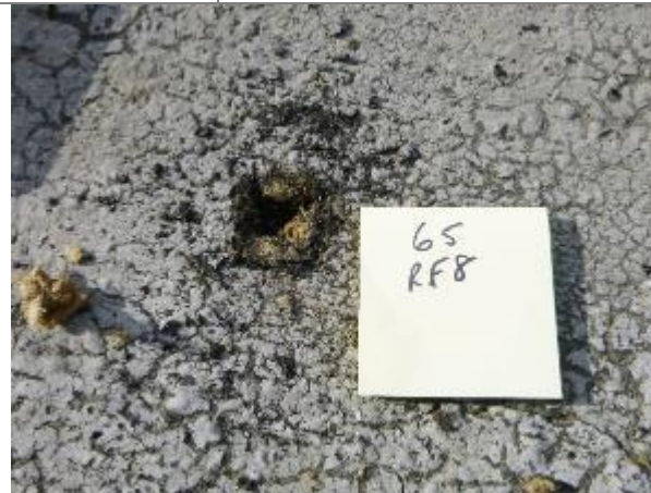
Photo #70 HA-65, silver and black built-up asphaltic roofing
