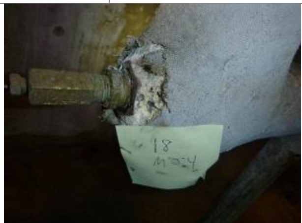
Photo #24 HA-18, gray cold and hot water pipe mudded joint fitting
