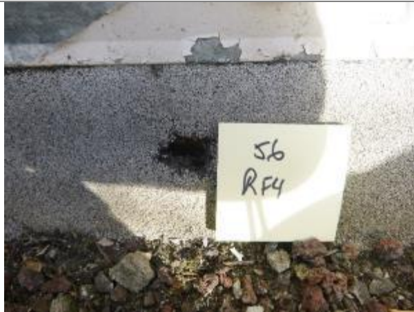
Photo #61 HA-56, gray rolled-on flashing with black tar
