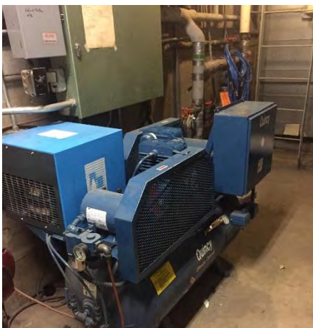
Photo #11 View of an air compressor in the mechanical room.
