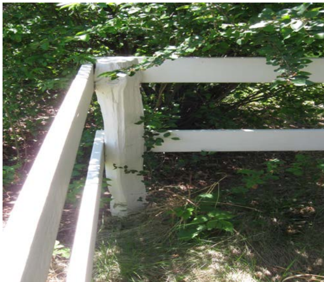
3-8. Example of hand hewn wooden fence posts supporting the fence on the east and south property boundaries.
