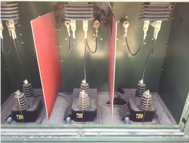
Damaged Metering Cabinet
