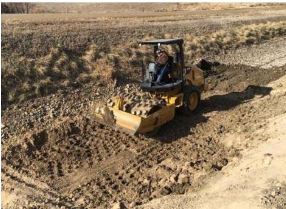
*Compacting the clay in the bottom of the Boulder Feeder Canal.*
