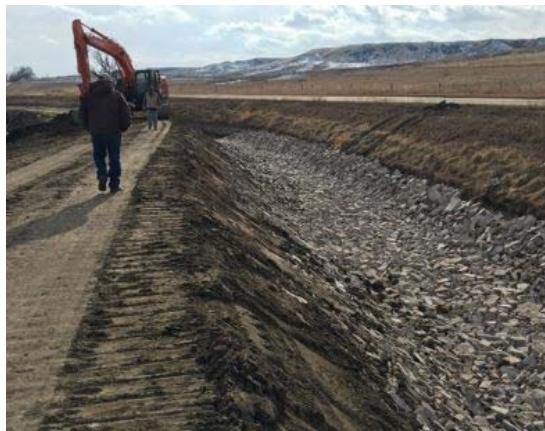
*Placement of rock to protect the compacted clay.*
