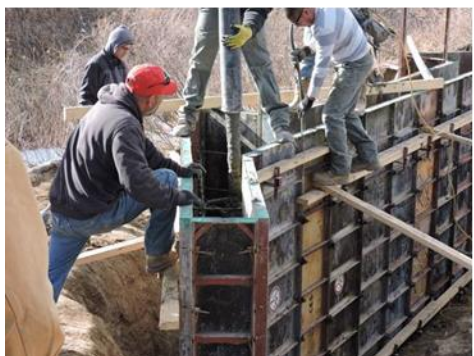
Pouring the North Bridge abutment – trail segment 10b, south of W. US 34 underpass
