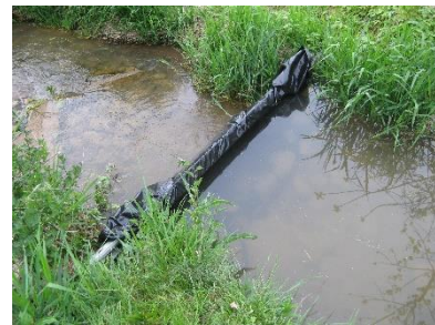
Tarp and ladder to dam water.
