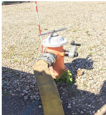
Fig. 15 – Hydrant ready to be charged.
