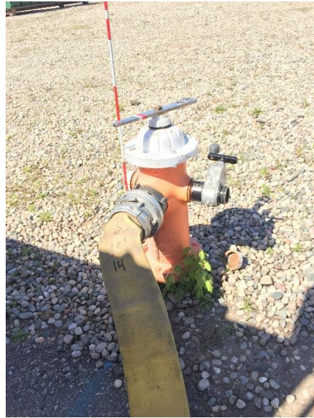
Fig. 6 – Hydrant ready to be charged.
