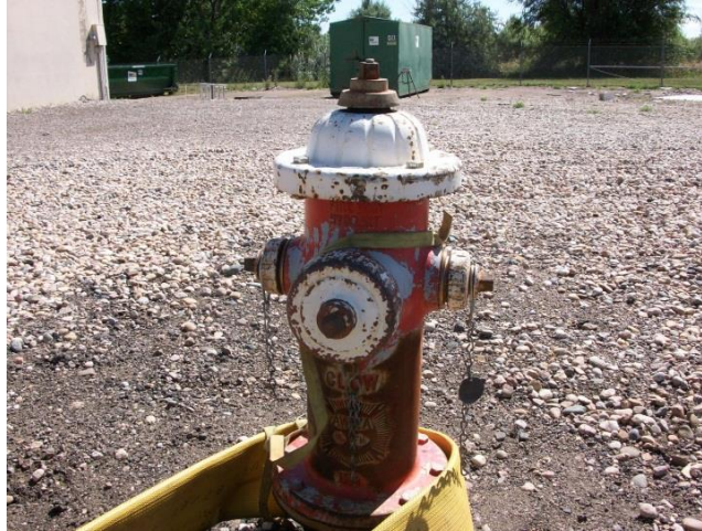
Fig. 4 Hydrant with LDH wrapped.
