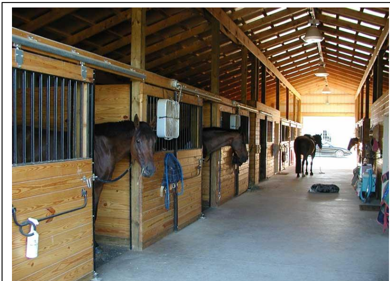
Figure 1: Unprotected trusses, potential heavy fire loading, unknown hazards, locking mechanisms, trip hazards, and frightened, dangerous animals.
