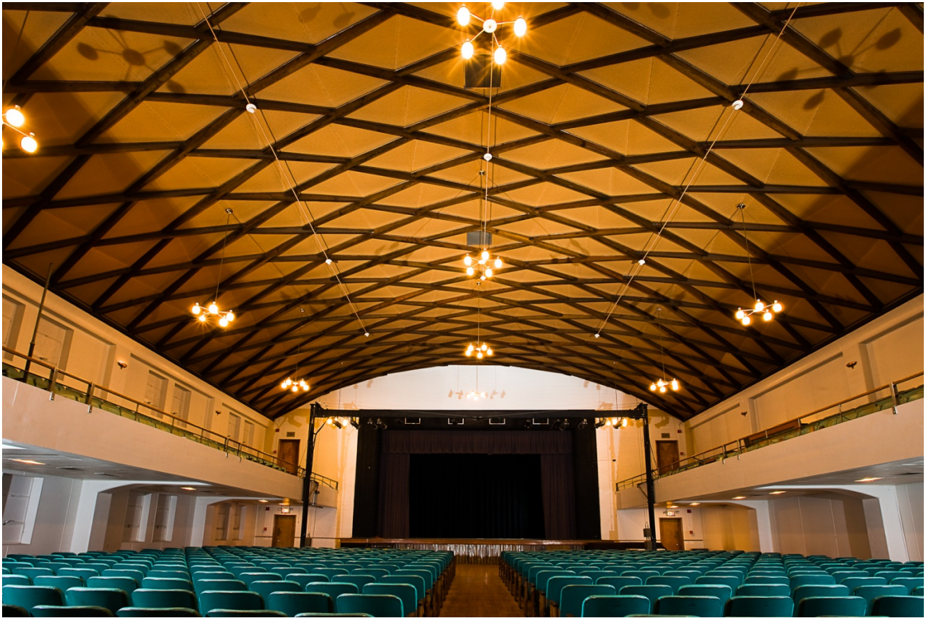
Figure 7: The Pulliam Auditorium with the Lamella Truss Roof.
