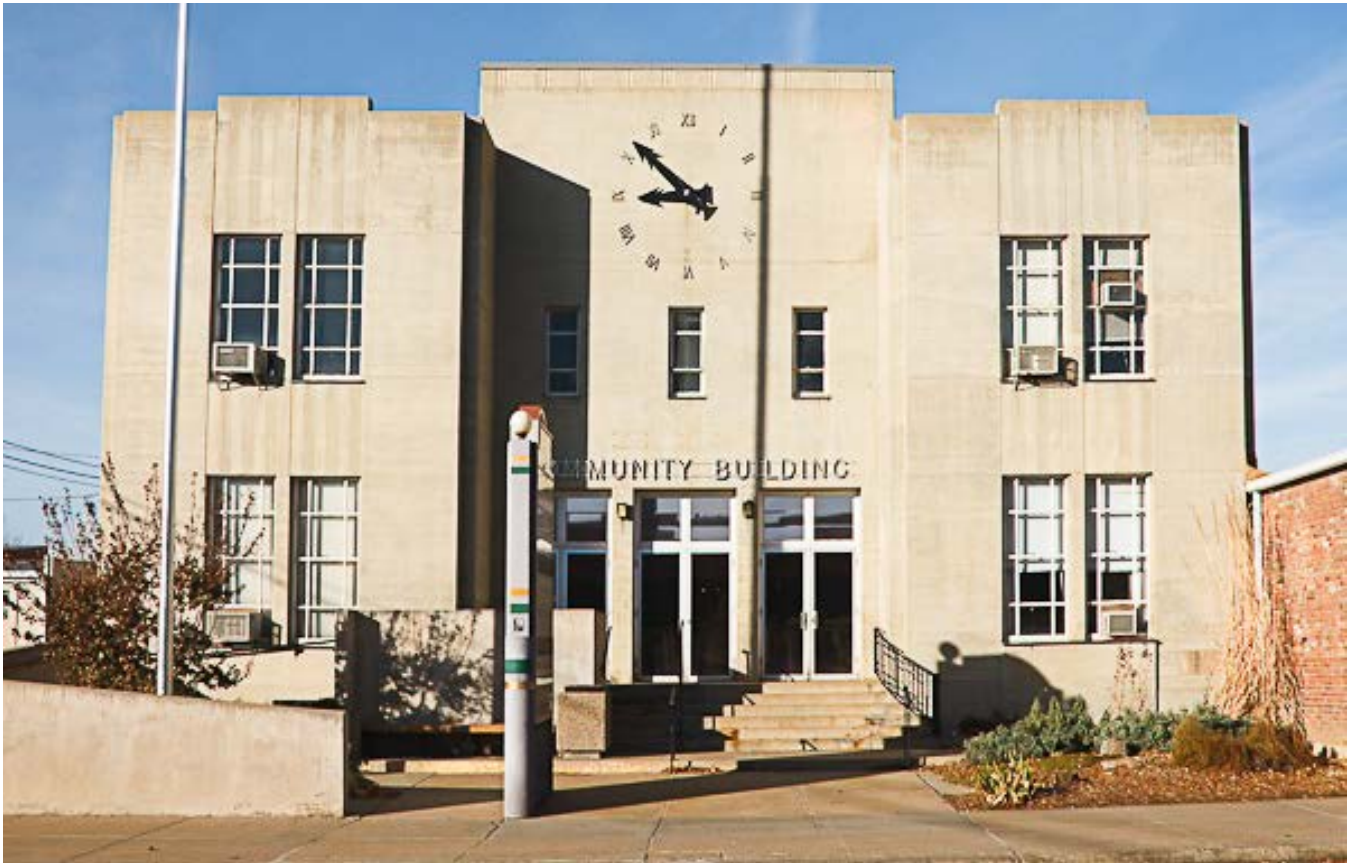
Figure 5: Pulliam Building Present Day. East (front) Elevation.
