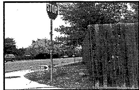
*This is a poorly designed intersection which does not give adequate visibility of on coming traffic.*
