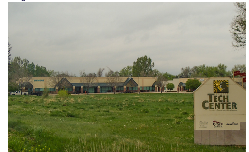
Loveland Tech Center northwest of US 287 & SH 60
