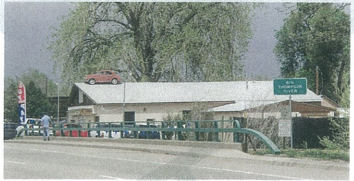
Big Thompson River Bridge
