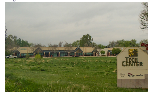
Loveland Tech Center northwest of US 287 & SH 60
