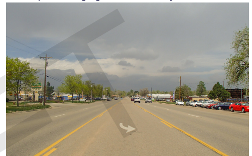
Roadway conditions in Zone 4
