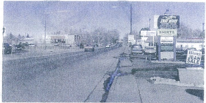
Multiple drive access points interrupt the sidewalk
