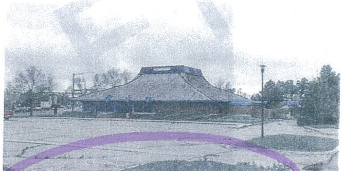
Vacant businesses do reflect the declining quality of the retail store mix
