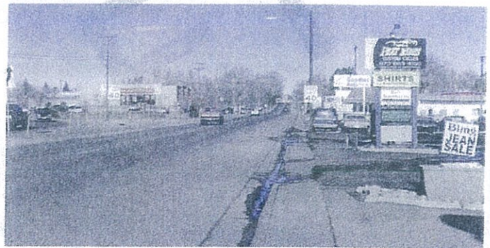
Multiple drive access points interrupt the sidewalk
