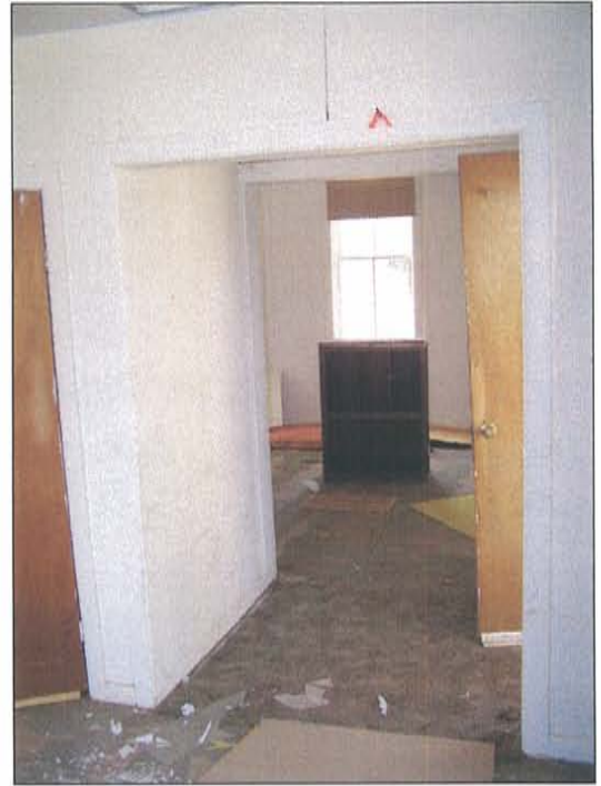
2007-HA-024 Milner Schwarz House September 21, 2007 Existing condition Image No. 077 Entry Hall Elevation
