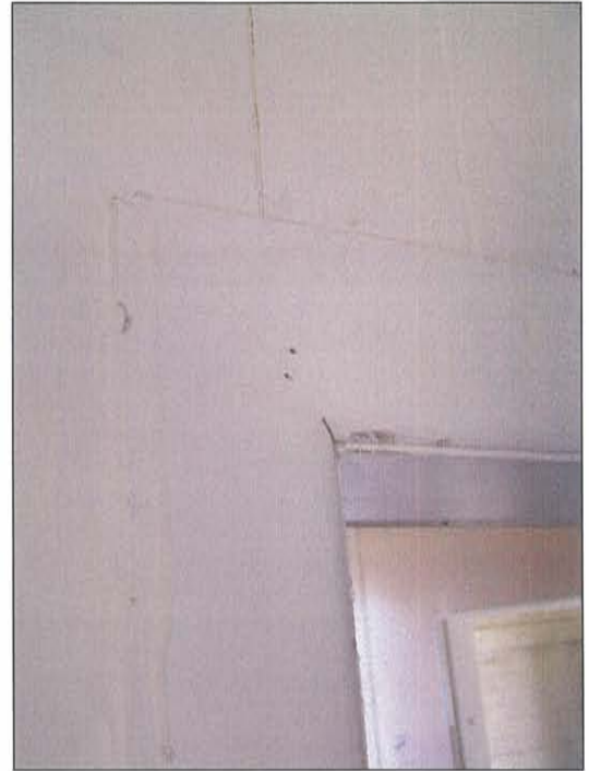
2007-HA-024 Milner Schwarz House September 21, 2007 Existing condition Image No. 133 Door Trim Detail
