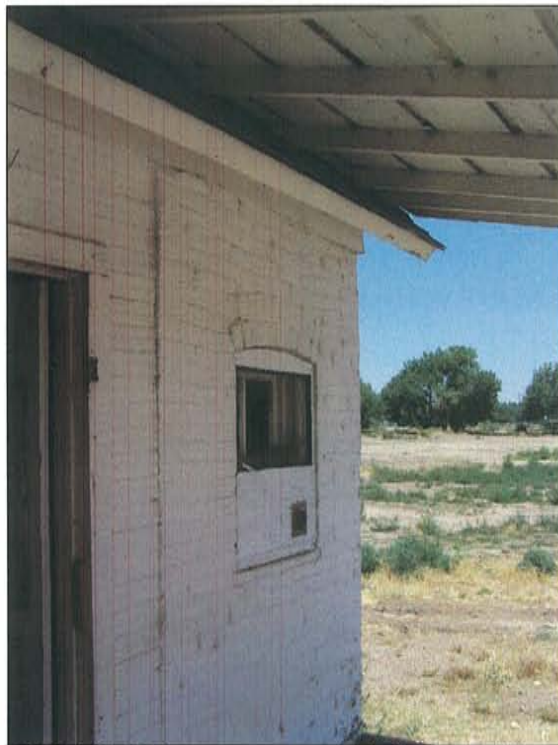
2007-HA-024 Existing condition Milner Schwarz House Image No. 032 September 21, 2007 Window Elevation
