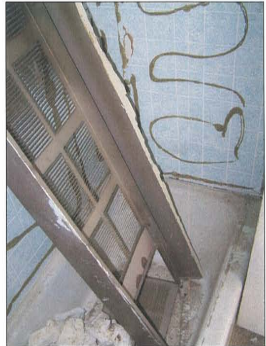
2007-HA-024 Existing condition Milner Schwarz House Image No. 087 September 21, 2007 Bathroom 103 Bathtub
