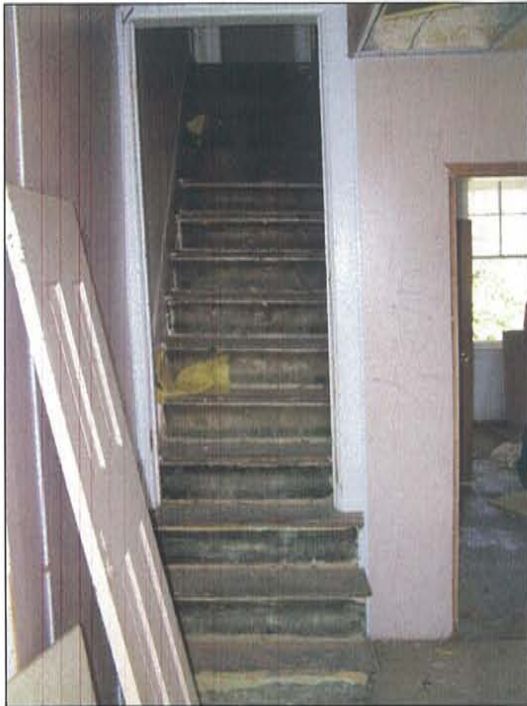
2007-HA-024 Milner Schwarz House September 21, 2007 Existing condition Image No. 094 Stair 109 Elevation
