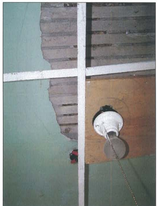
2007-HA-024 Milner Schwarz House September 21, 2007 Existing condition Image No. 155 Light Detail
