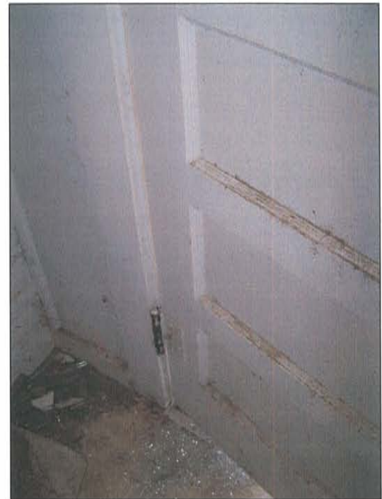
2007-HA-024 Milner Schwarz House September 21, 2007 Existing condition Image No. 135 Door Detail
