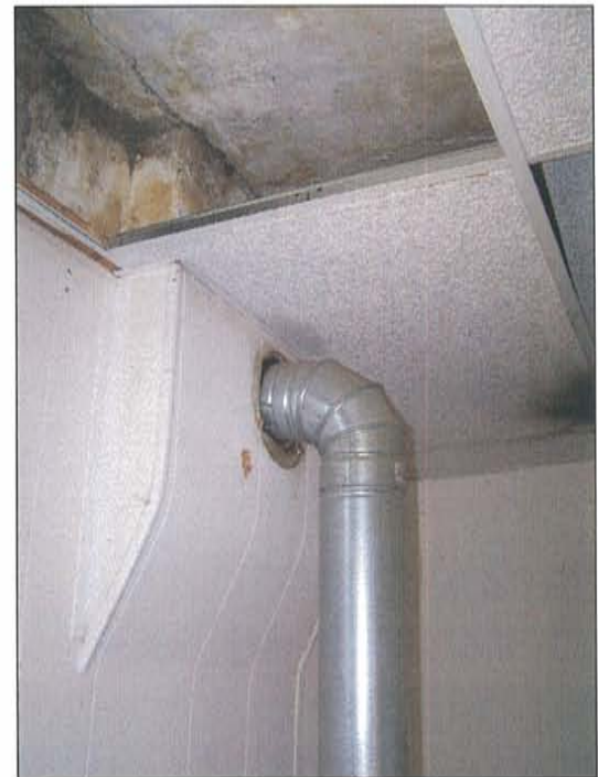
2007-HA-024 Existing condition Milner Schwarz House Image No. 093 September 21, 2007 Heater Vent Detail
