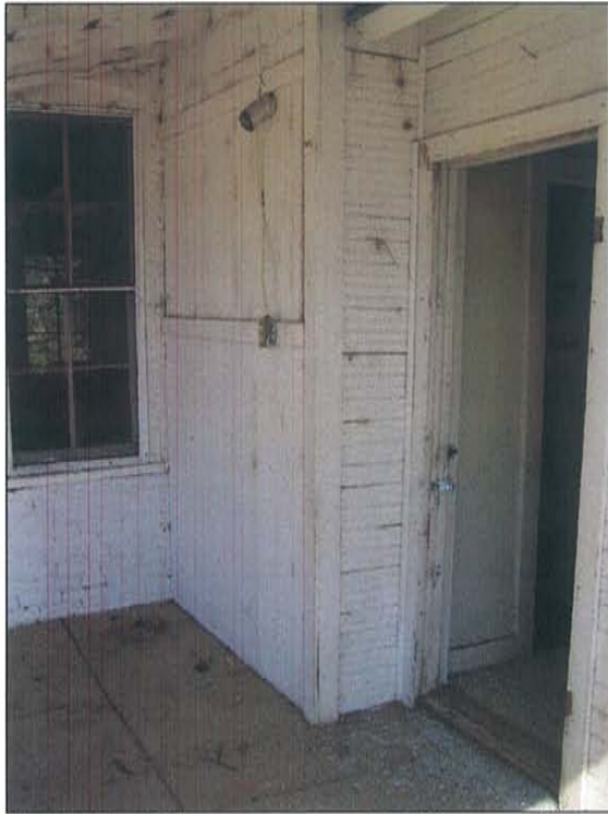
2007-HA-024 Existing condition Milner Schwarz House Image No. 030 September 21, 2007 Rear Door
