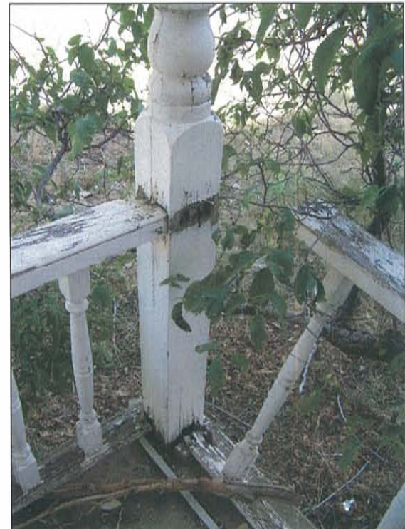
2007-HA-024 Existing condition Milner Schwarz House Image No. 020 September 21, 2007 Front Porch Railing
