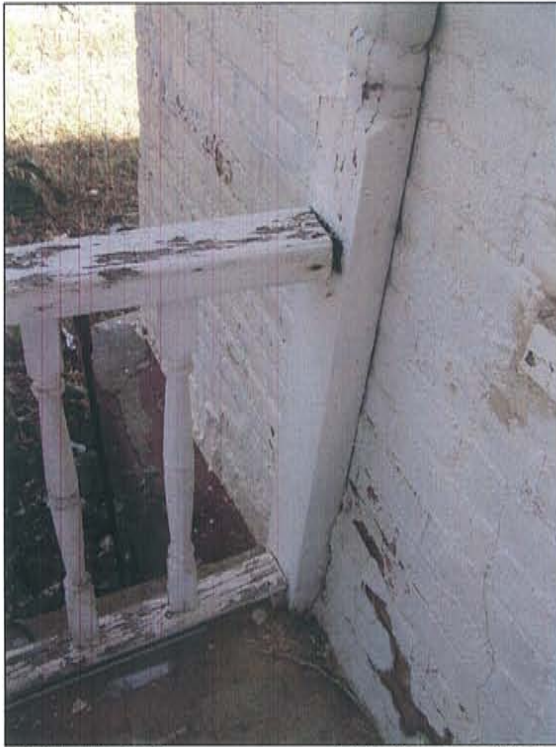
2007-HA-024 Existing condition Milner Schwarz House Image No. 017 September 21, 2007 Front Porch Railing
