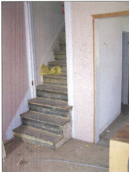
2007-HA-024 Milner Schwarz House September 21, 2007 Existing condition Image No. 096 Stair 109 Elevation
