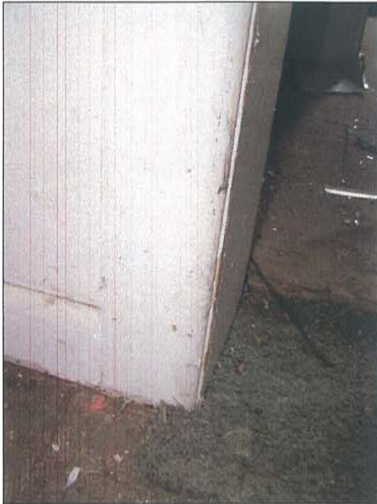
2007-HA-024 Milner Schwarz House September 21, 2007 Existing condition Image No. 132 Door Trim Detail
