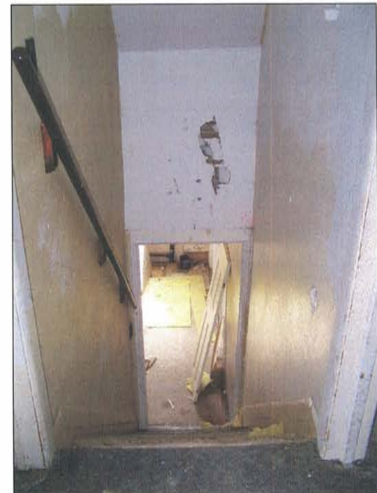
2007-HA-024 Milner Schwarz House September 21, 2007 Existing condition Image No. 097 Stair 203 Elevation
