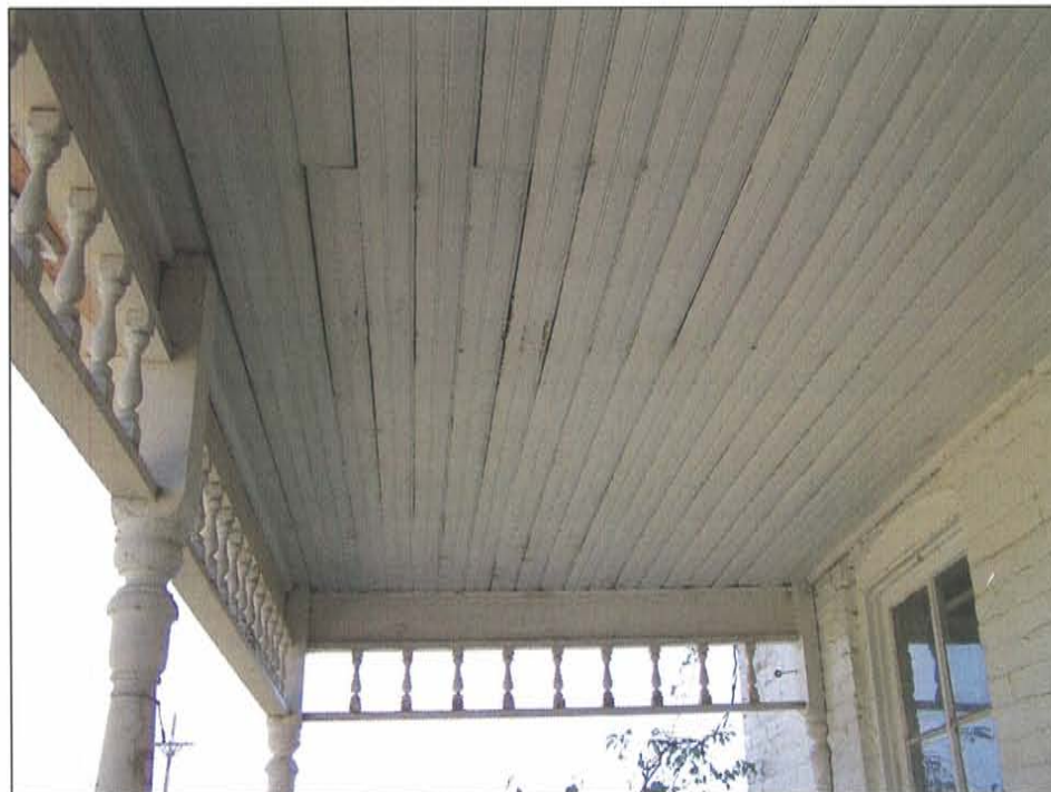
Existing condition Image No. 012 Front Porch Ceiling Detail
