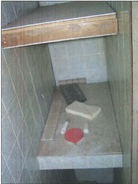
2007-HA-024 Existing condition Milner Schwarz House Image No. 086 September 21, 2007 Bathroom 103 Shelves
