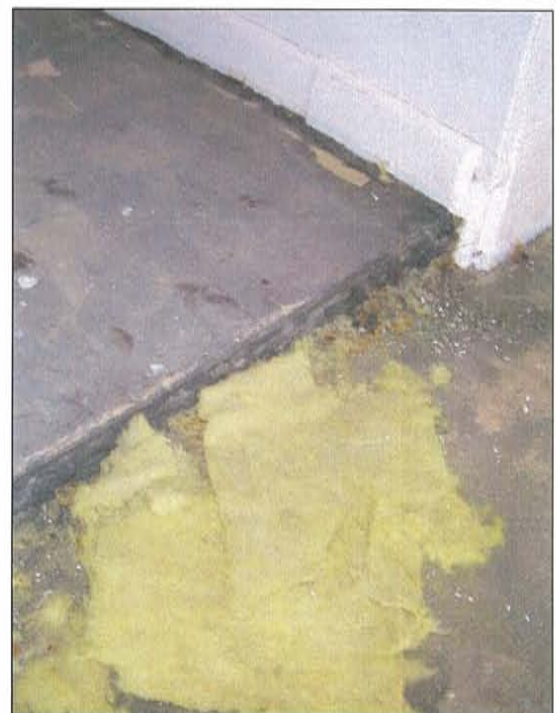
2007-HA-024 Milner Schwarz House September 21, 2007 Existing condition Image No. 112 Floor Detail (Upper Floor)
