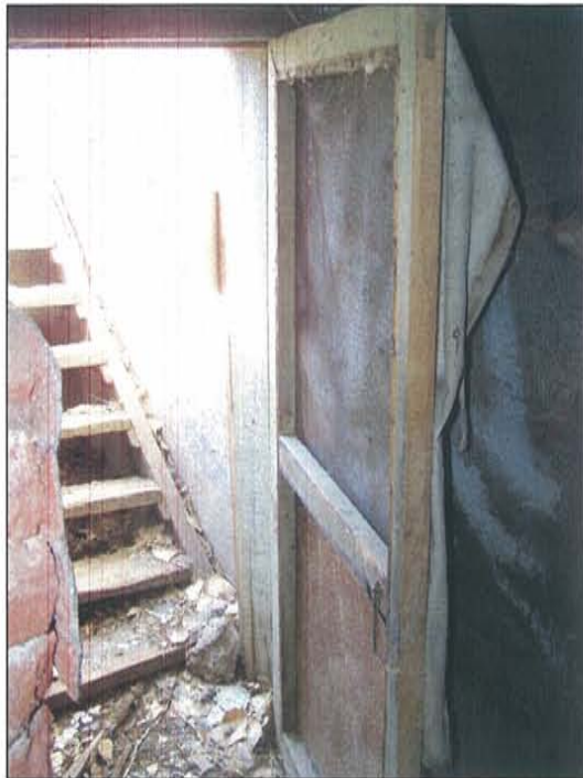
2007-HA-024 Existing condition Milner Schwarz House Image No. 106 September 21, 2007 Cellar Stairs & Door
