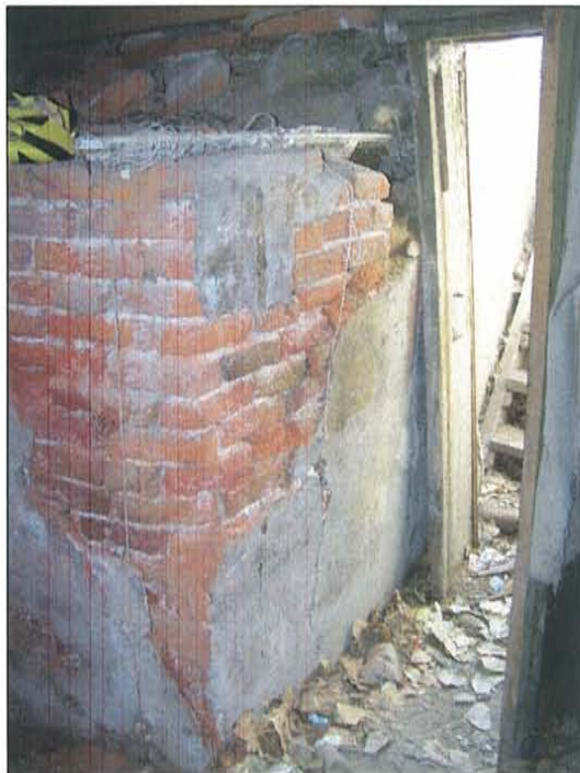
2007-HA-024 Existing condition Milner Schwarz House Image No. 108 September 21, 2007 Basement Detail
