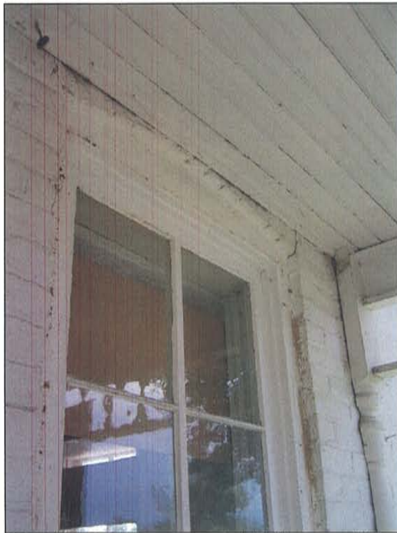
2007-HA-024 Existing condition Milner Schwarz House Image No. 056 September 21, 2007 Window Head Detail
