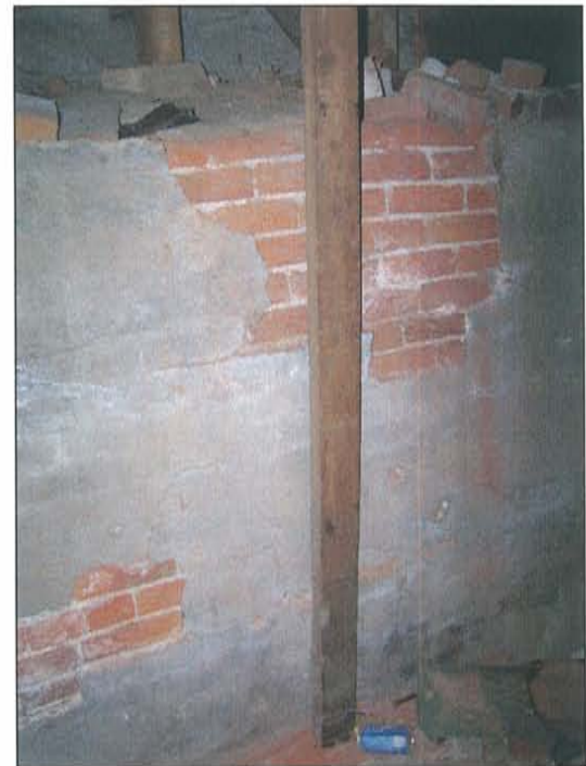
2007-HA-024 Existing condition Milner Schwarz House Image No. 109 September 21, 2007 Basement Detail
