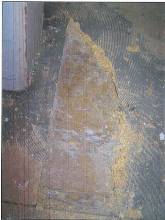
2007-HA-024 Milner Schwarz House September 21, 2007 Existing condition Image No. 111 Floor Detail (Upper Floor)
