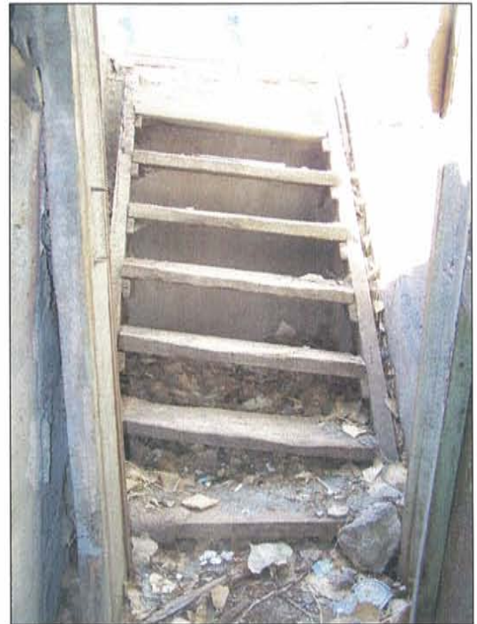
2007-HA-024 Existing condition Milner Schwarz House Image No. 107 September 21, 2007 Cellar Stairs
