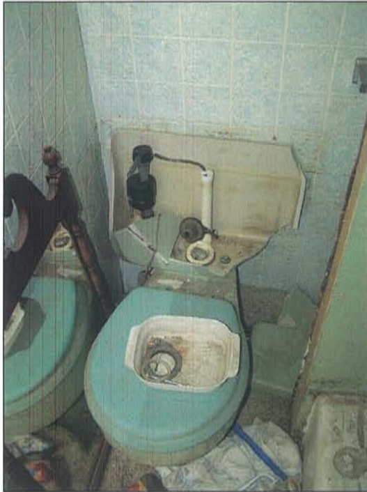
2007-HA-024 Existing condition Milner Schwarz House Image No. 084 September 21, 2007 Bathroom 103 Toilet
