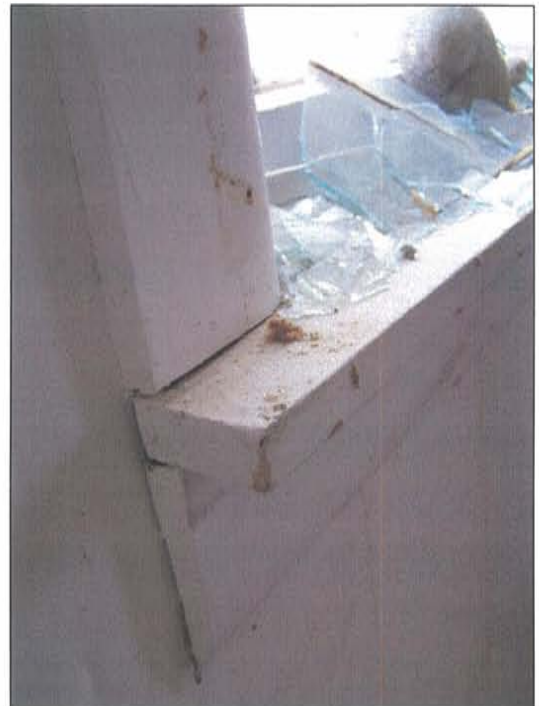
2007-HA-024 Milner Schwarz House September 21, 2007 Existing condition Image No. 153 Window Sill Detail
