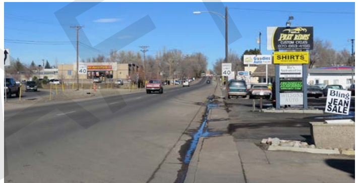
Multiple drive access points interrupt the sidewalk
