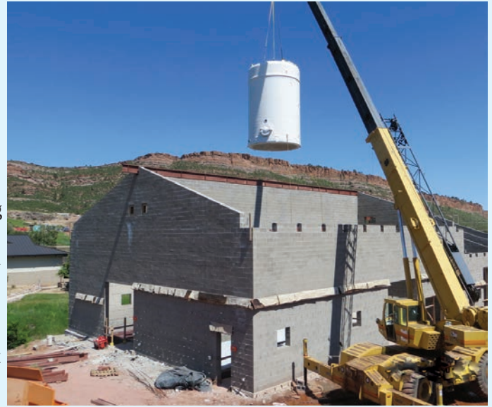
The new West Chemical building at the treatment plant will house a 22,500 gallon tank that holds the solution used water disinfection.
