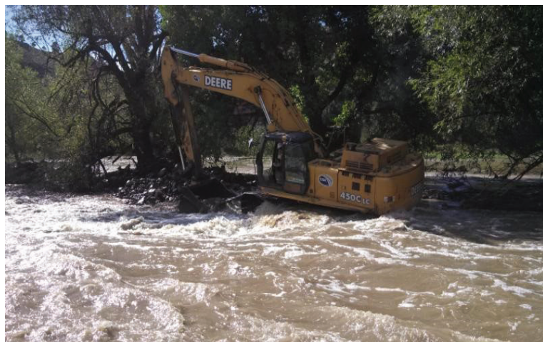
An excavator works to dig out the original river channel following the September 2013 Flood.
