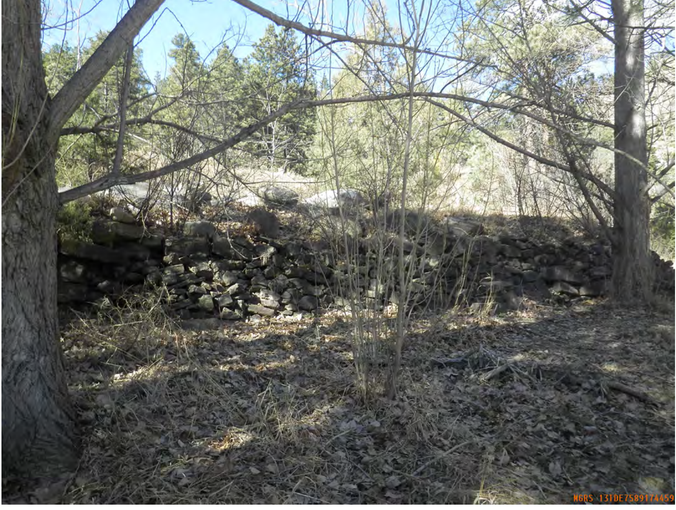
12. CCC era dry-stacked stone wall.
