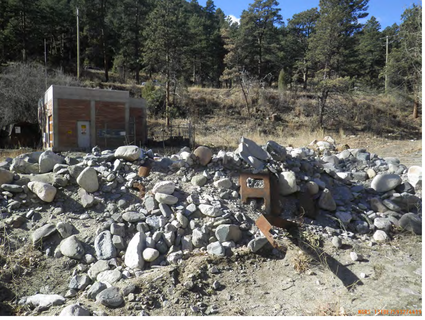
20. Hydroelectric turbines buried in mud and debris with former power plant building beyond.
