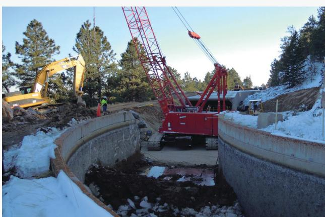
Crews install Pole Hill Canal box culvert sections.
