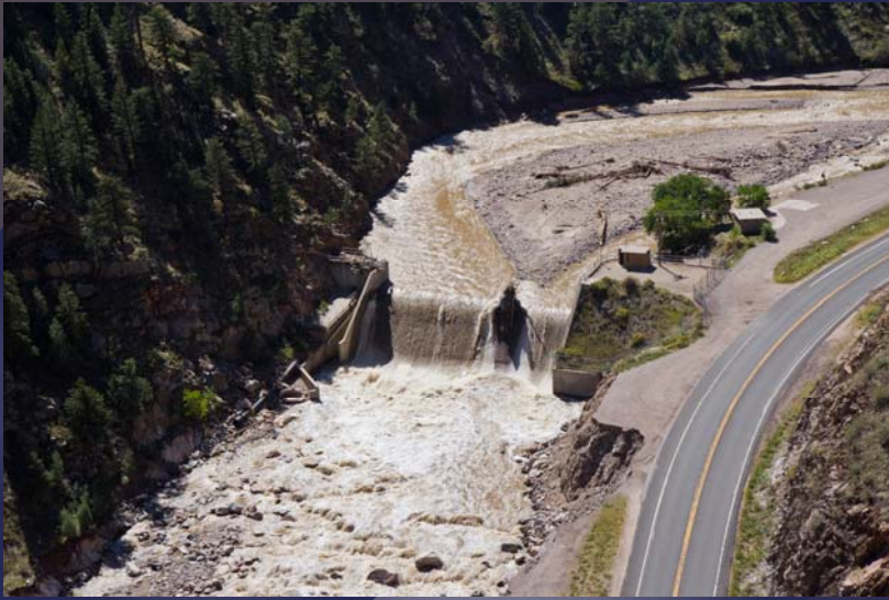
Idylwilde Dam post 2013 Flood Concern about dam stability, reservoir filled with silt, sand, cobble and boulders
