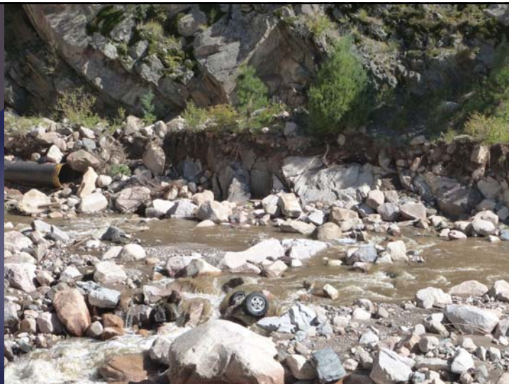
Pipeline post 2013 Flood Downstream from Idylwilde Dam, Exposed pipe with portion missing
