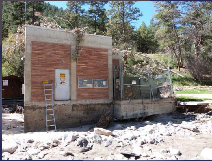
Power Plant post 2013 Flood Erosion around foundation
