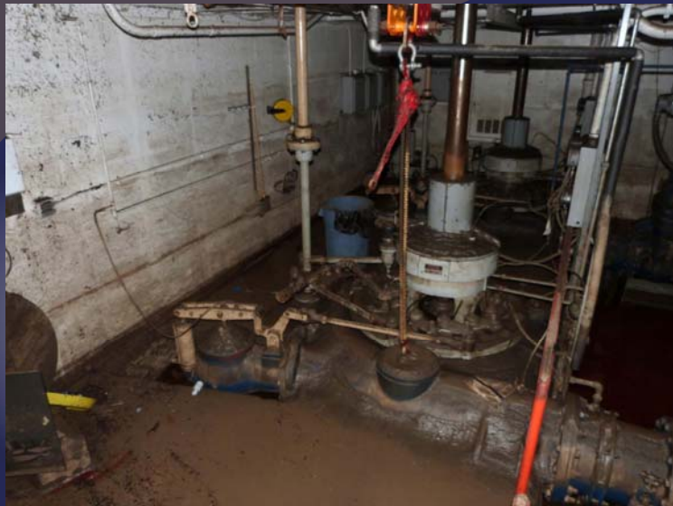
Power Plant post 2013 Flood Inside is filled with muck
