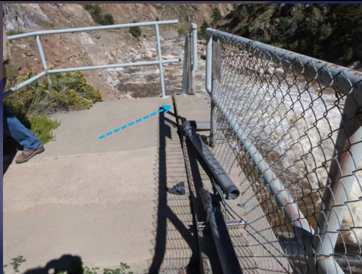
Idylwilde Dam post 2013 Flood Disconnected pipe and concrete separation
