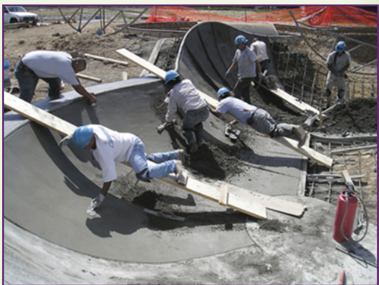
Concrete Work on Bowl-Shaped Skate Area
