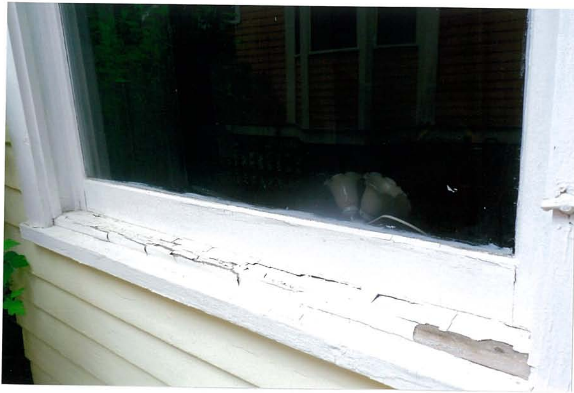
South Side window No storm window Rotted sill
