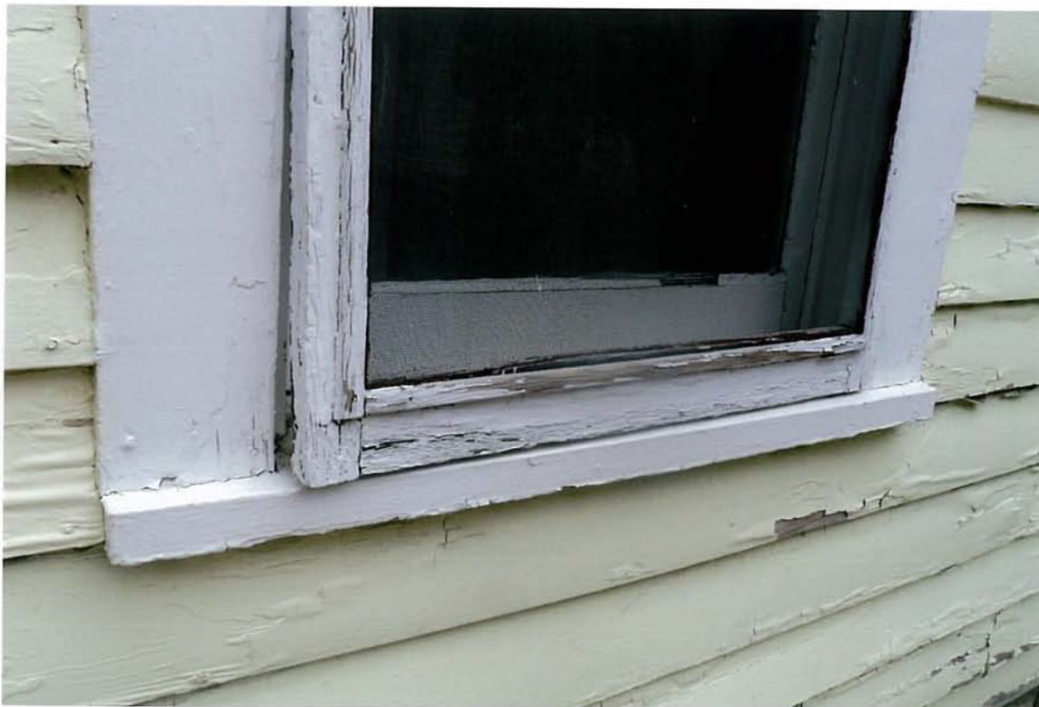
ROTTED WINDOW - North side ROTTED STORM WINDOW - Doesn't fit.
