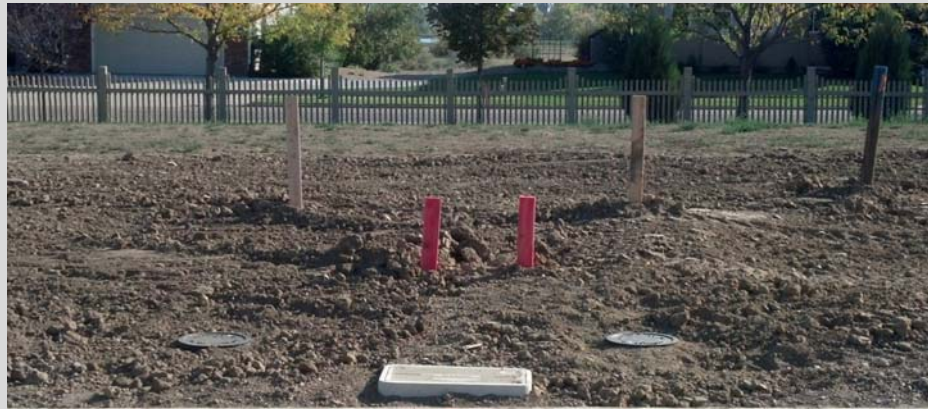
Final grade: Conduit stub is marked by red painted posts.
