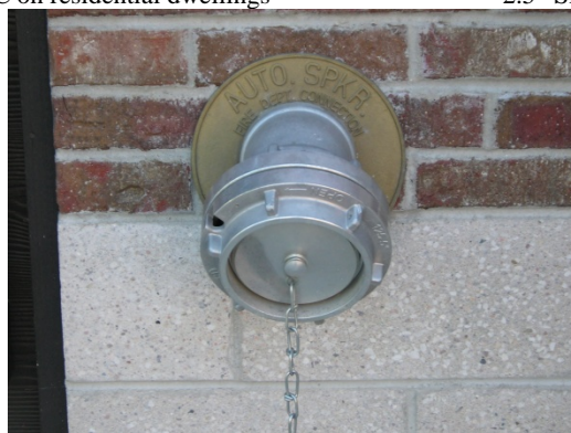
5" FDC on combination Standpipe/Sprinkler System
