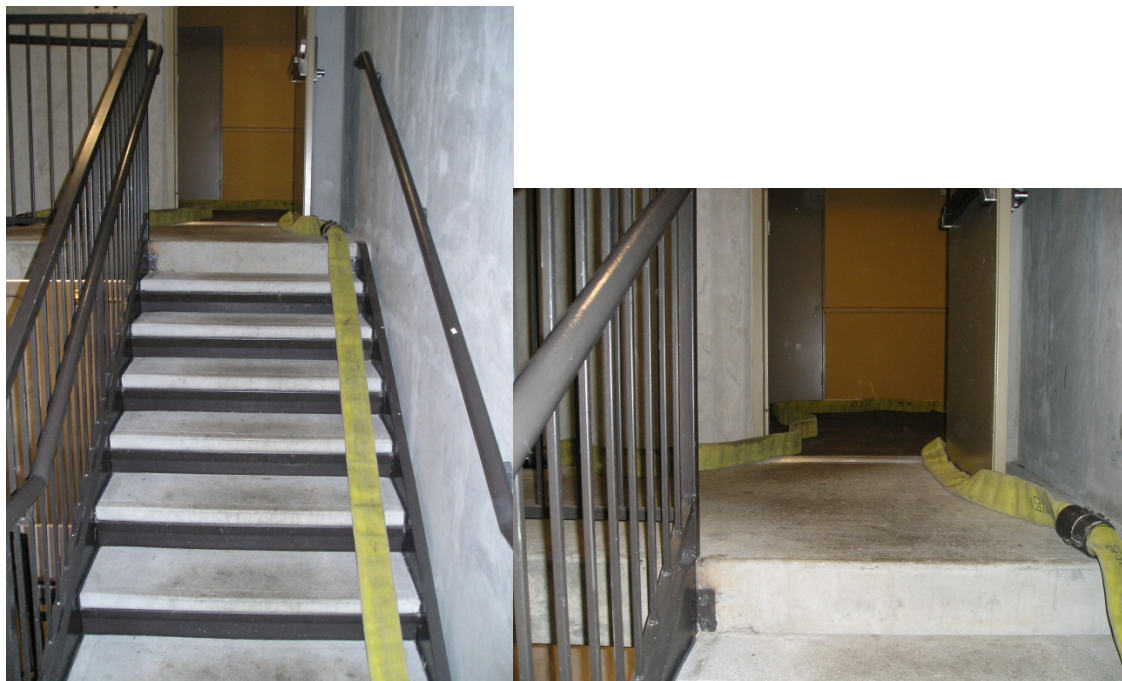
Using the space provided on the floor below to dress the hose
