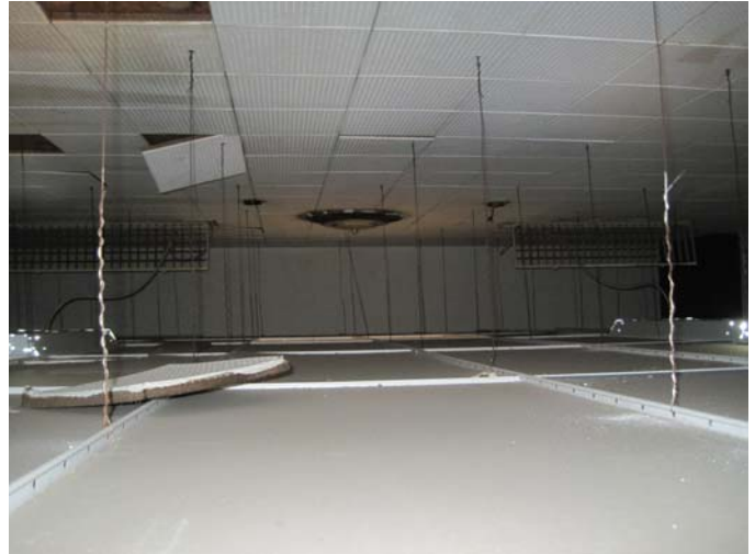
LEL0969 HISTORIC DIFFUSER ABOVE SUSPENDED CEILING IN FIRST FLOOR CONFERENCE ROOM
