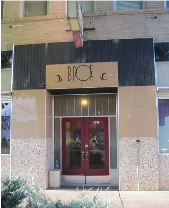
LEL9352 EXTERIOR STOREFRONT FINISHES, FURRED AND FACE APPLIED AT SOUTH GROUND LEVEL
