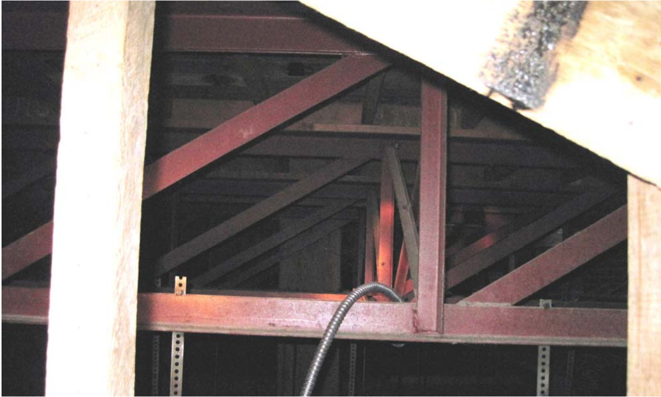
LEL7748 STEEL TRUSSES, WOOD FRAMING, AND STEEL SUPPORT STRAPS ABOVE LODGE ROOM
