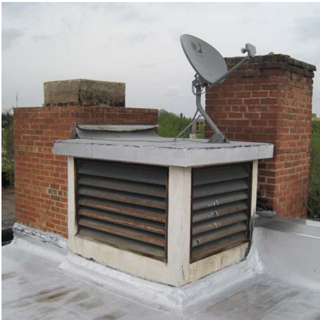
LEL7724 NORTHEAST CORNER VENT CHASE AND CHIMNEY (ACTIVE BOILER FLUE)
