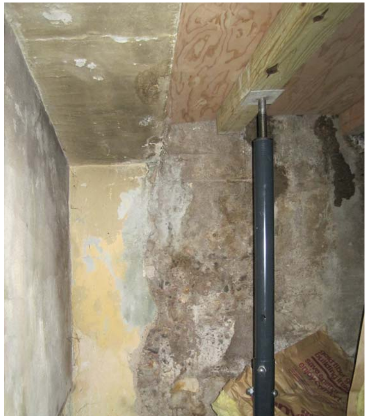
LEL7420 HISTORIC PLASTERED ARCH (AT LEFT), BRACING, AND SUB-SIDEWALK CONCRETE (AT RIGHT)
