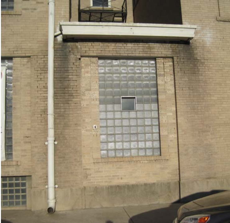
LEL9343 MASONRY DAMAGE FROM OVERFLOW AT EDGES OF FIRST FLOOR ROOF BELOW LIGHT WELL
