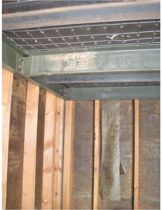
LEL7744 WOOD AND STEEL STRUCTURAL SYSTEM OF ROOFTOP ELEVATOR ENCLOSURE
