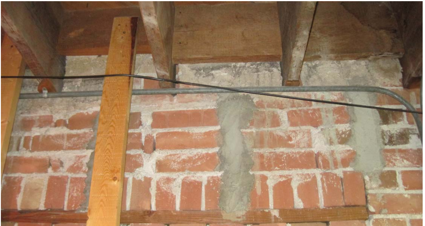
LEL7464 BRICK FOUNDATION WALL IN FAN ROOM SHOWING RETROFITTED FLOOR JOIST CONFIGURATION
