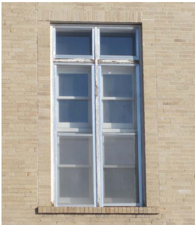
LEL1058 WEST ELEVATION LODGE ROOM STACKED PAIRED DOUBLE HUNG WINDOWS
