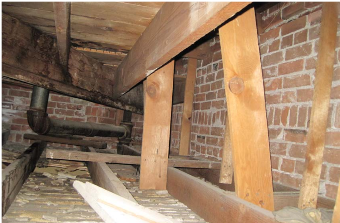
LEL7821 ROOF FRAMING, INTERNAL ROOF DRAIN, AND CEILING FRAMING SOUTH OF LIGHT WELL AT SOUTH ROOF NEAR WEST WALL, CAMERA FACING WEST
