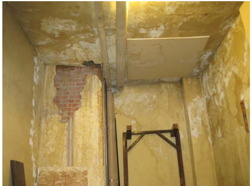
LEL7565 PLASTER FINISHES IN DRESSING ROOM (DAMAGED BY LEAKING OF COOLING UNIT IN MECHANICAL ROOM ABOVE)
