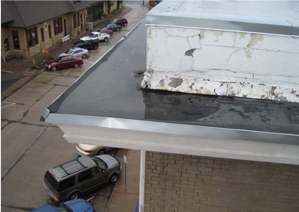
LEL7707 SOUTHWEST CORNER OF NORTH ROOF AT LIGHT WELL SHOWING SHEET METAL PARAPET CAP, PARAPET, MEMBRANE COVERED INTEGRAL GUTTER, SHEET METAL CORNICE, AND BRICK MASONRY
