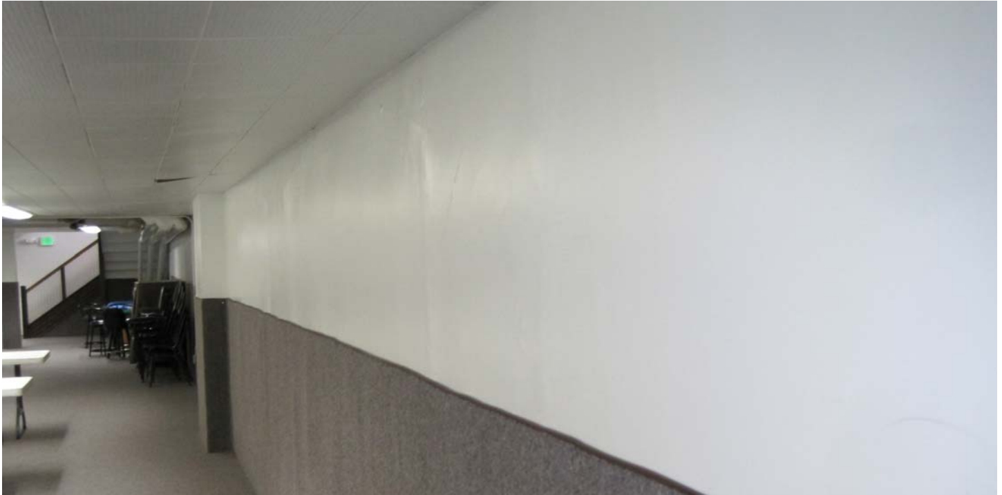
LEL7409 VIEW LOOKING SOUTH ALONG WEST BASEMENT WALL SHOWING GHOSTING OF ARCHED OPENINGS
