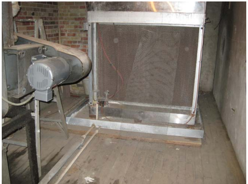
LEL1026 CLOSER VIEW OF BASE OF COOLING UNIT, AT LOCATION OF NORTHEAST CORNER LEAKS ABOVE DRESSING ROOM
