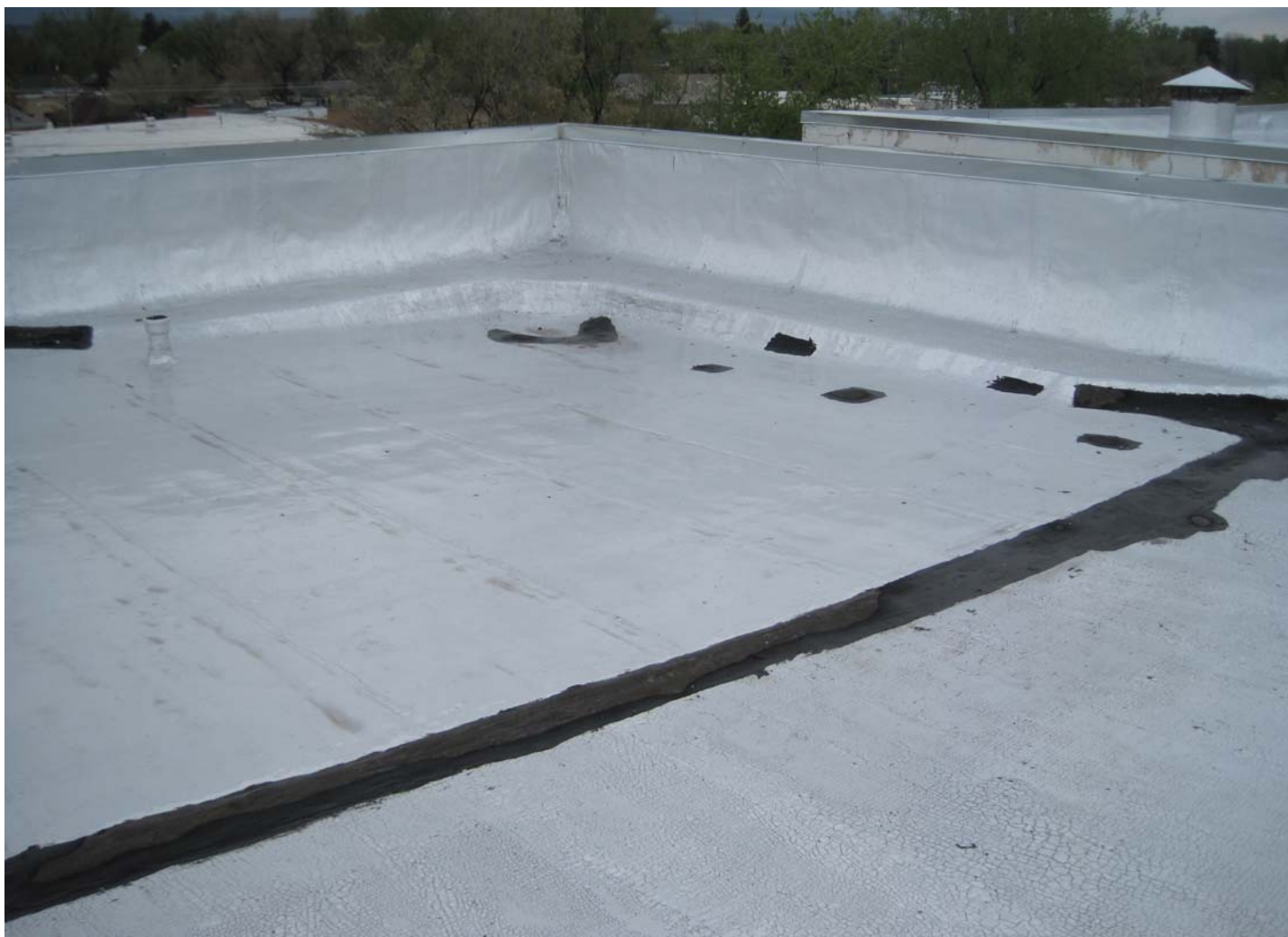
LEL7705 AREA OF PONDING, INTERIOR DRAIN, AND ROOF LEAKS (NOTE MULTIPLE PATCHES) AT NORTHWEST CORNER OF SOUTH ROOF, SOUTH OF LIGHT WELL
