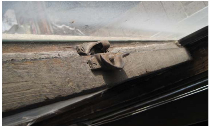
LEL0993 SASH LOCK ON ORIGINAL SOUTH WINDOW
