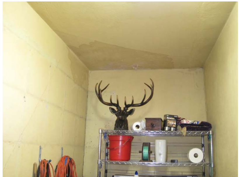
LEL7617 CLOSER VIEW OF STORAGE ROOM WATER DAMAGE AND ADJACENT FINISHES
