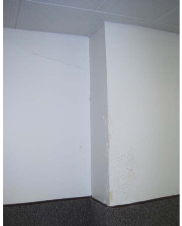
LEL7413 BUBBLED PAINT ON BASEMENT WEST WALL
