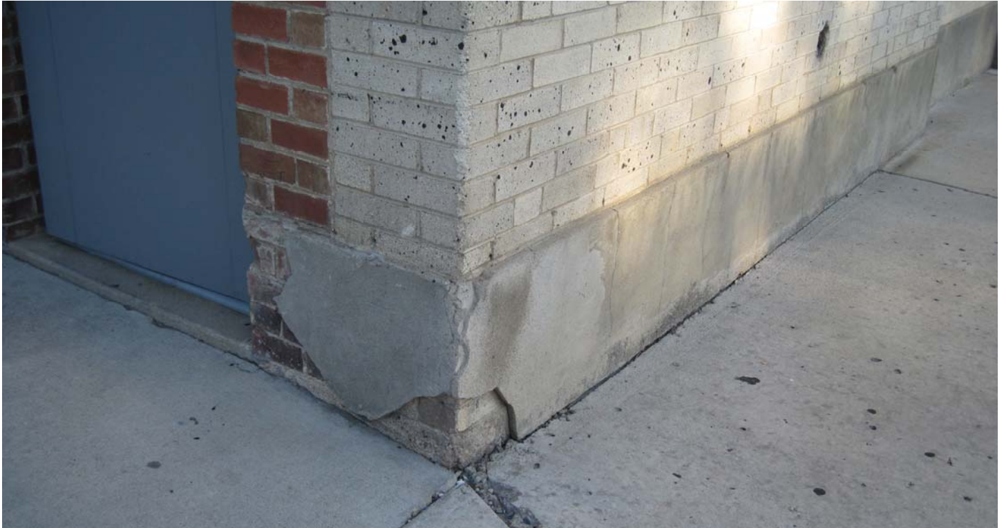
LEL9333 NORTHWEST CORNER VIEW SHOWING CONCRETE PARGING ALONG TOP OF FOUNDATION
