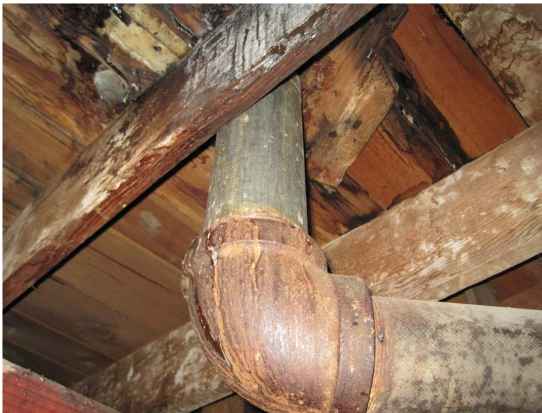
LEL7798 WATER DAMAGE AND INTERNAL ROOF DRAIN NEAR WEST END OF SOUTH ROOF, SOUTH OF LIGHT WELL
