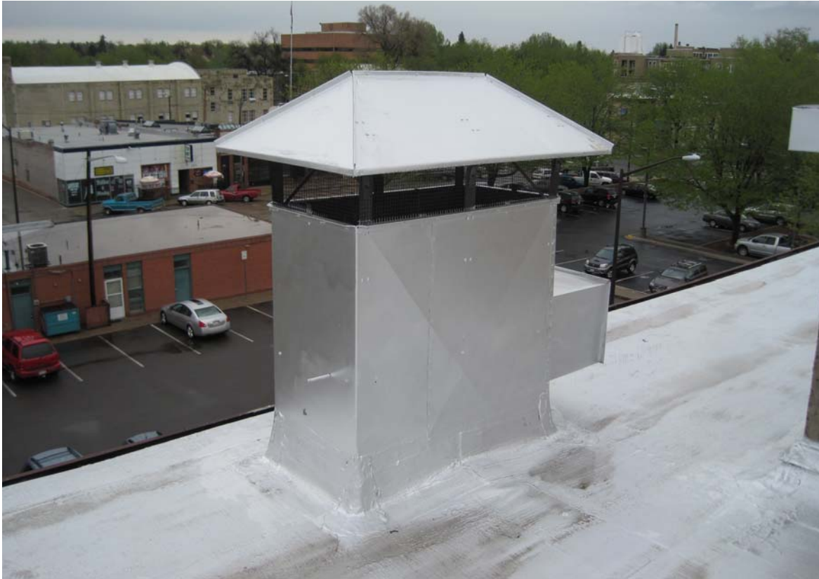
LEL7732 VENTILATION CHASE AT CENTRAL NORTH END OF ROOF
