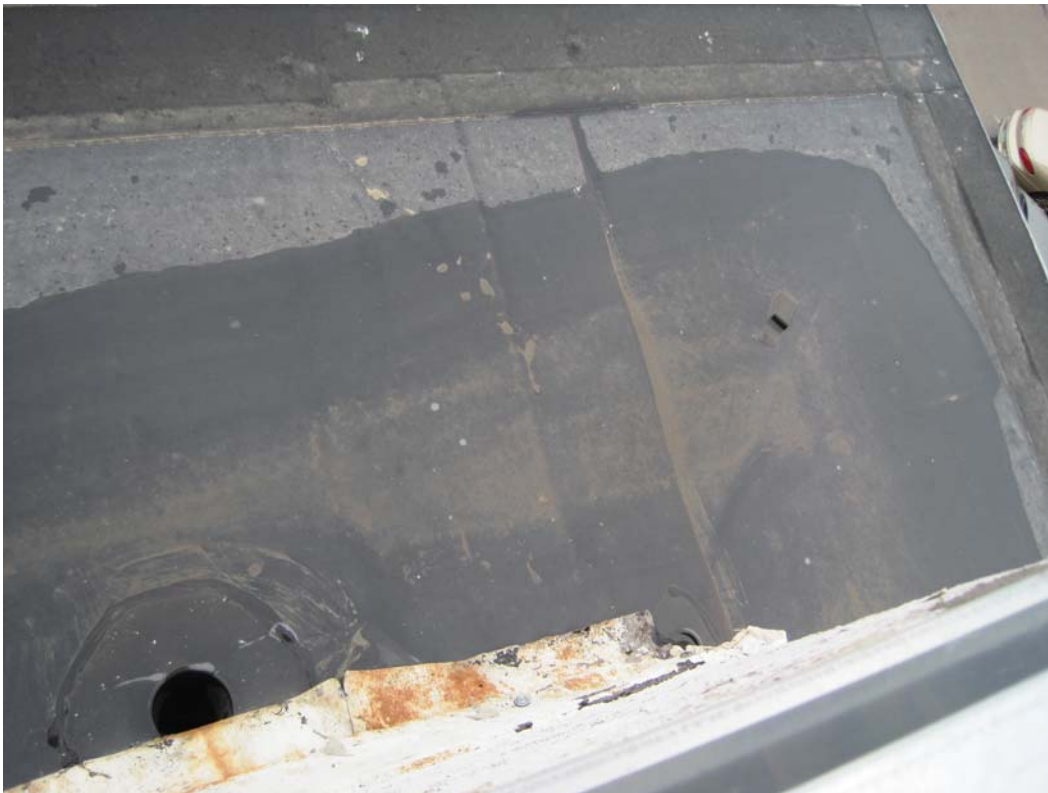
LEL7706 MEMBRANE COVERED INTEGRAL GUTTER AT WEST SIDE OF NORTHWEST CORNER OF SOUTH ROOF
