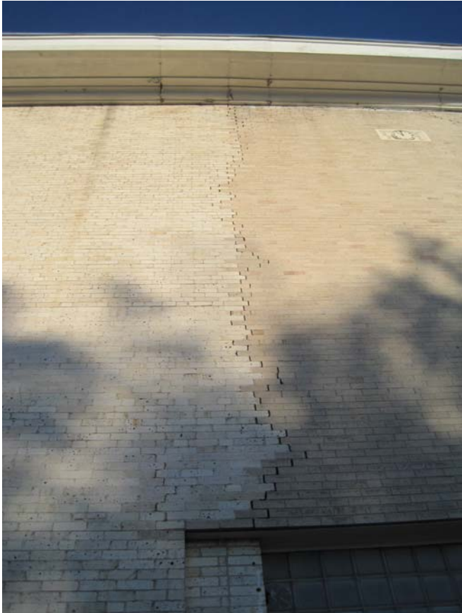
LEL9336 OPEN TOOTHING AT NORTH ADDITION INTERFACE WITH OLDER MASONRY
