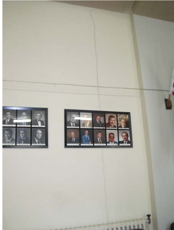
LEL7606 PLASTER FRACTURE ON EAST WALL OF LODGE ROOM, POSSIBLY LOCATED AT HISTORIC LIGHT WELL LOCATION
