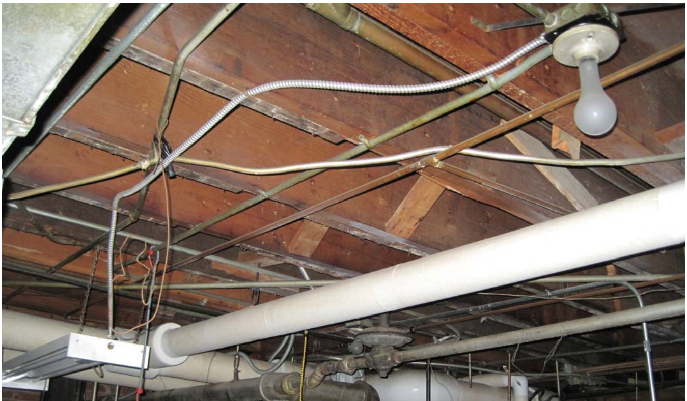
LEL7364 FLOOR JOISTS AND BRACING IN BASEMENT BOILER ROOM
