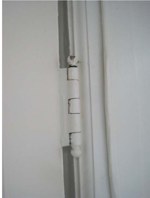
LEL7326 TYPICAL HISTORIC BASEMENT DOOR BALL TIPPED HINGE
