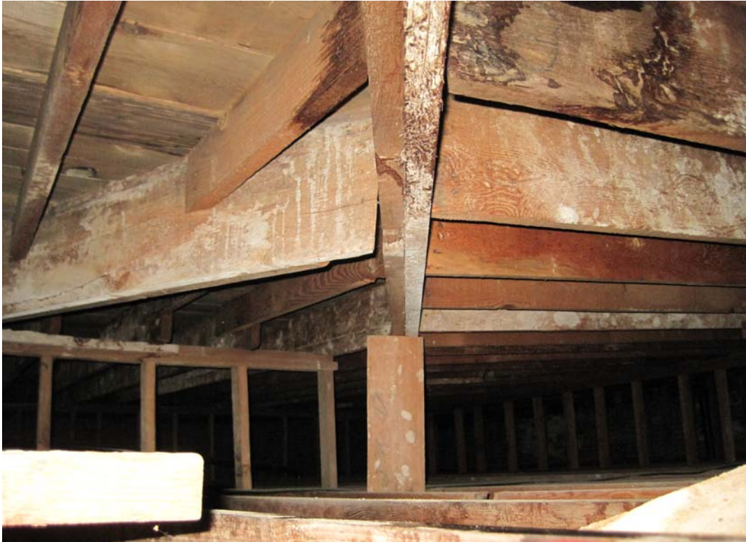
LEL7800 VALLEY BEAM AND ROOF FRAMING OF SOUTH ROOF NEAR LIGHT WELL, CAMERA FACING SOUTHEAST
