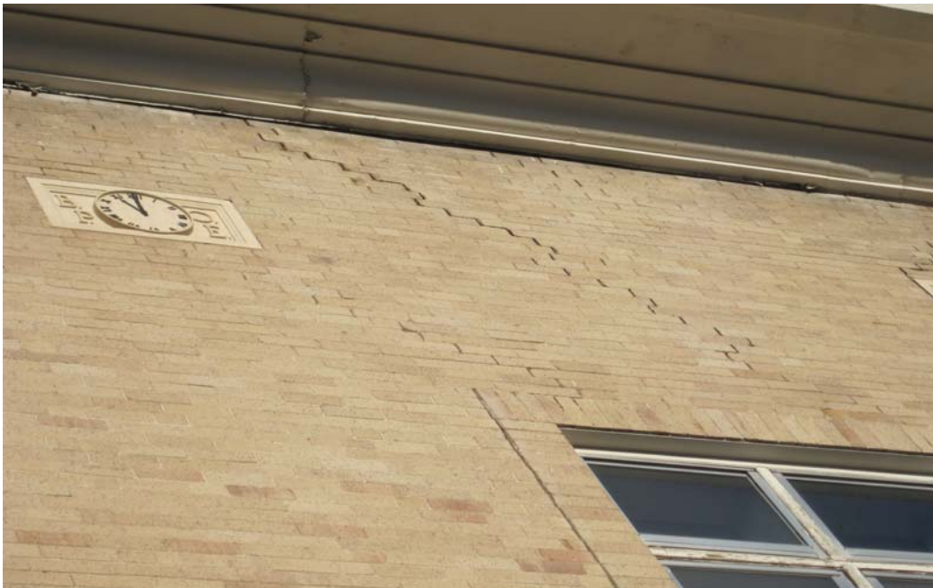
LEL9335 IN-PLANE CORBEL PATTERN CRACKING ABOVE NORTH END OF NORTH WINDOW ON WEST ELEVATION
