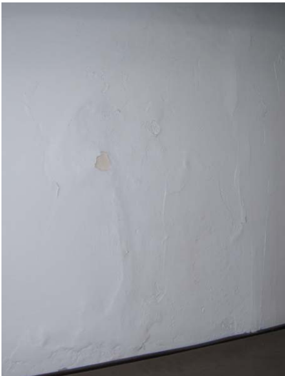
LEL7417 PATCHED SPALLED CONCRETE AT WEST FOUNDATION WALL
