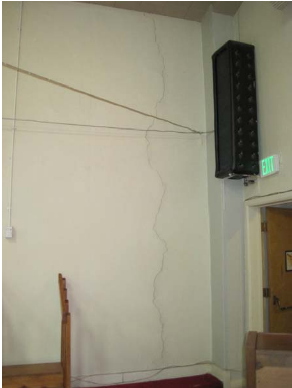
LEL7596 PLASTER FRACTURE ON WEST WALL OF LODGE ROOM THAT COINCIDES WITH BRICK MASONRY GAP SHOWN IN PHOTO #LEL9336
