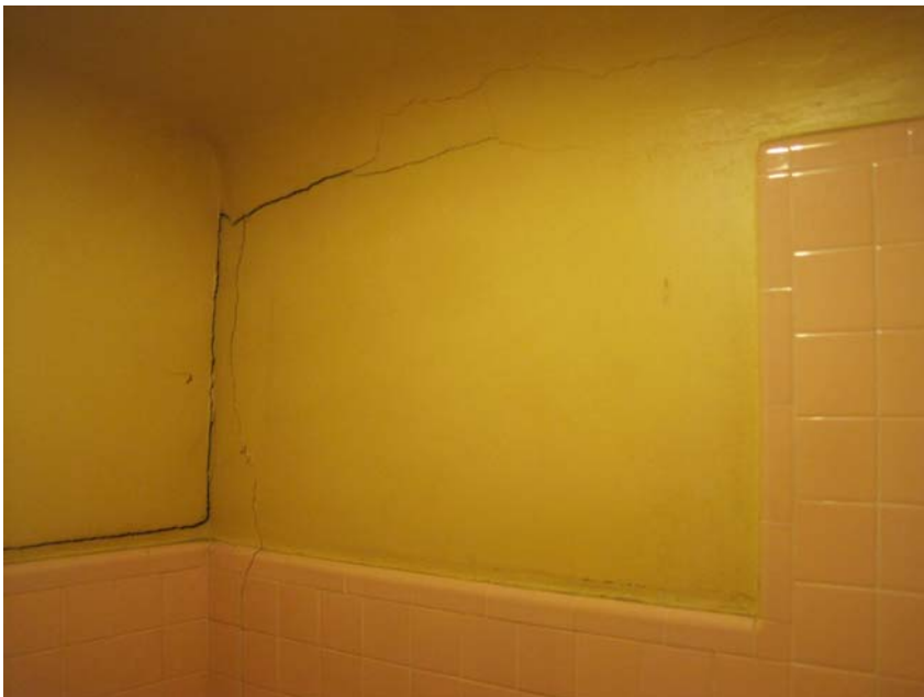
LEL7520 DRAMATIC PLASTER AND TILE FRACTURES AT NORTHEAST CORNER OF SHOWER STALL LOCATED AT SOUTH END OF BASEMENT MEN'S RESTROOM
