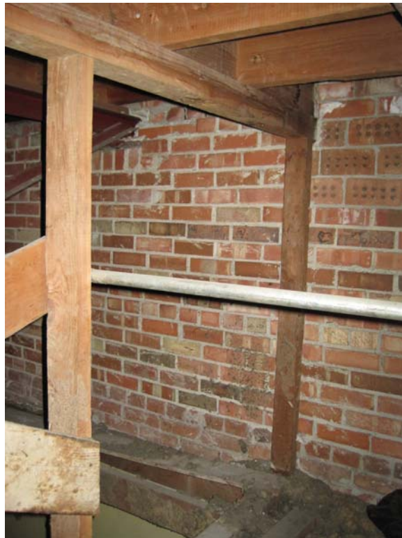
LEL7754 STEEL TRUSS (IN BACKGROUND) BEARING ON WEST BRICK MASONRY WALL
