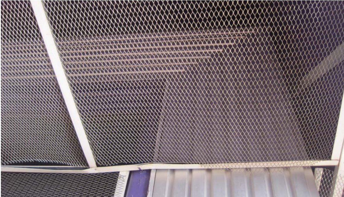
LEL1061 VIEW OF MILL FINISH ALUMINUM TRIM OF WEST DOOR EXTENDING INTO SCREENED AWNING SPACE
