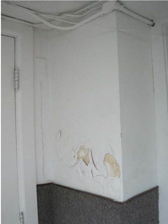
LEL7538 BUBBLED PAINT ON FOUNDATION WALL SOUTH OF ELEVATOR DOOR
