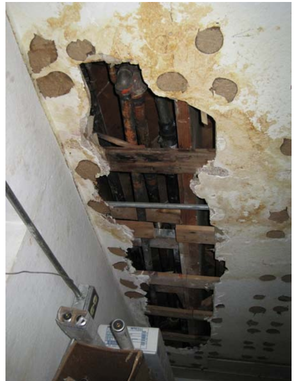
LEL7483 DAMAGED CEILING PLASTER IN LARGE STORAGE ROOM
