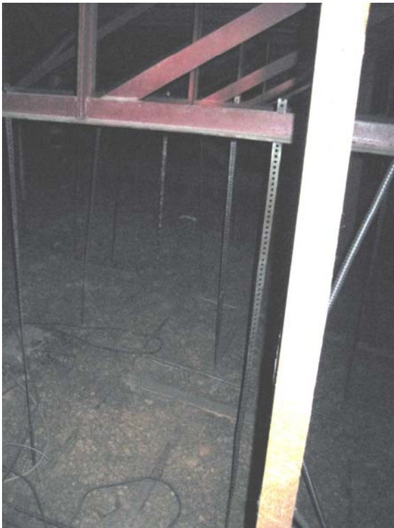
LEL7749 STEEL TRUSSES WITH STRAPS SUPPORTING LODGE ROOM CEILING
