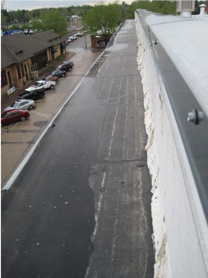
LEL7715 COVERED INTEGRAL GUTTER OF SHEET METAL CORNICE ON WEST ELEVATION
