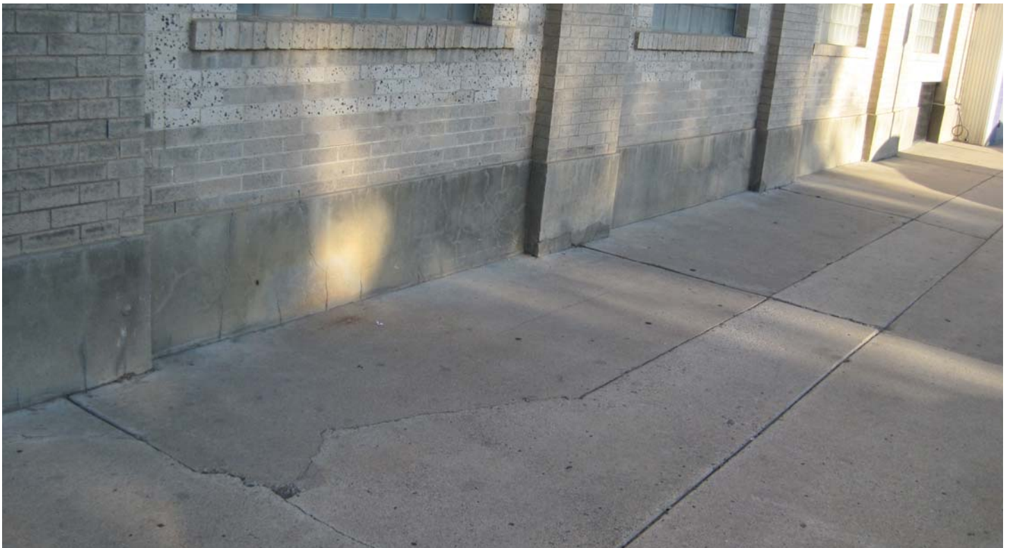
LEL9342 WEST ELEVATION NEAR NORTHWEST CORNER SHOWING CONCRETE INFILL AT LOCATION OF HISTORIC GLASS PAVERS ABOVE VAULTS ADJACENT TO AND PREVIOUSLY OPEN TO FOUNDATION WALL
