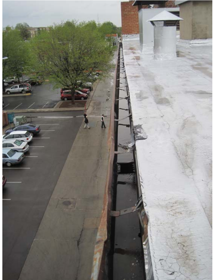
LEL7726 BOX GUTTER AT NORTH EDGE OF NORTH ROOF
