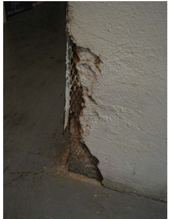
LEL7526 DAMAGE AT BASE OF NORTH STORAGE ROOM WALL EXPOSING METAL LATH BENEATH PLASTER
