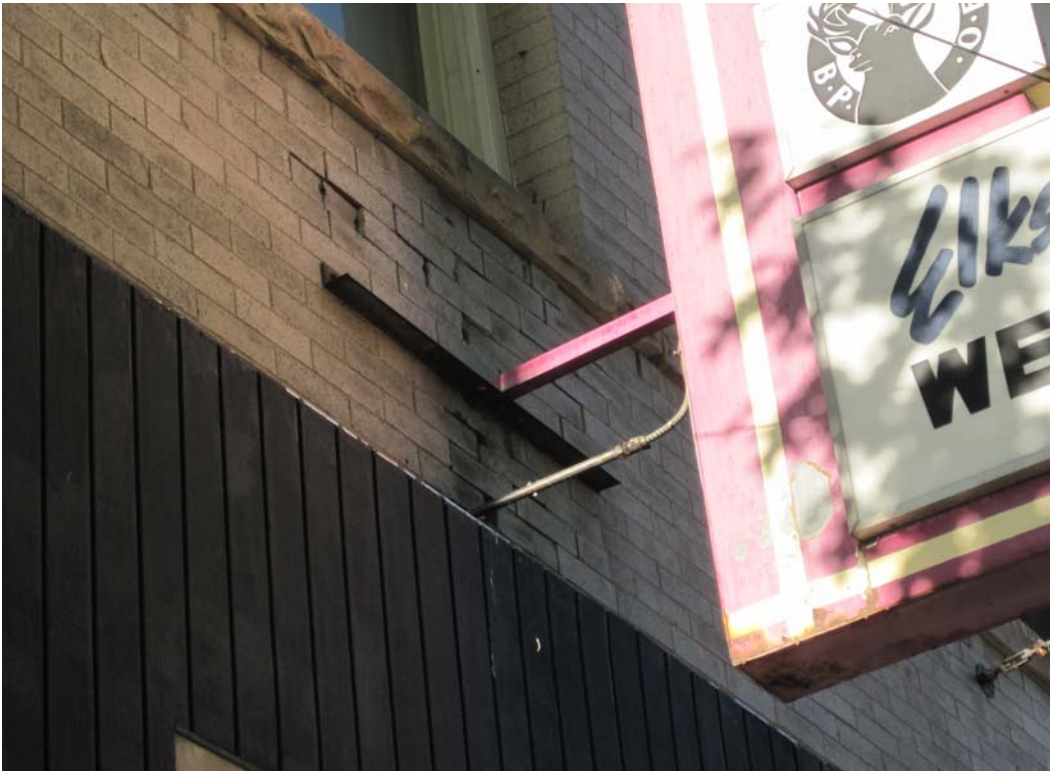
LEL9354 BRICK DAMAGE FROM PRIOR SIGN ATTACHMENT ON SOUTH ELEVATION ABOVE STOREFRONT
