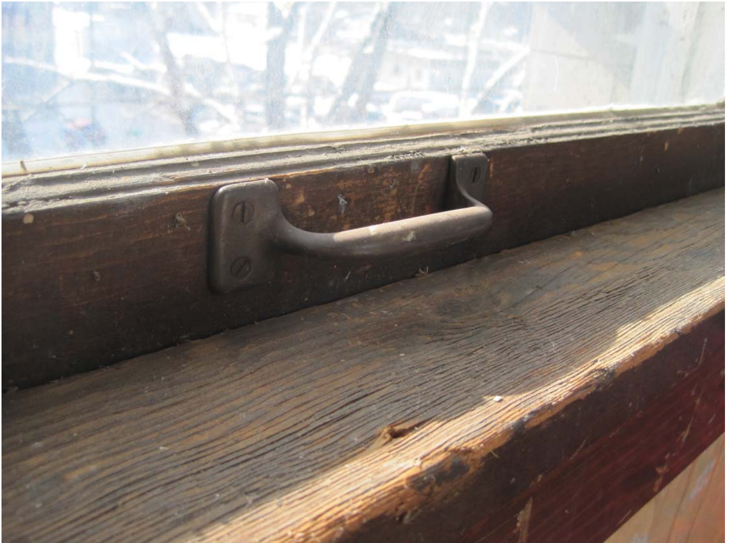
LEL0995 SASH PULL ON ORIGINAL SOUTH WINDOW, AND ADJACENT ORIGINAL FINISHES CONDITION
