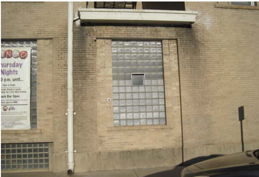
LEL9343 CORNICE WITH INTEGRAL GUTTER ON ROOF BELOW LIGHT WELL (NOTE EROSION AND BRICK STAINING)
