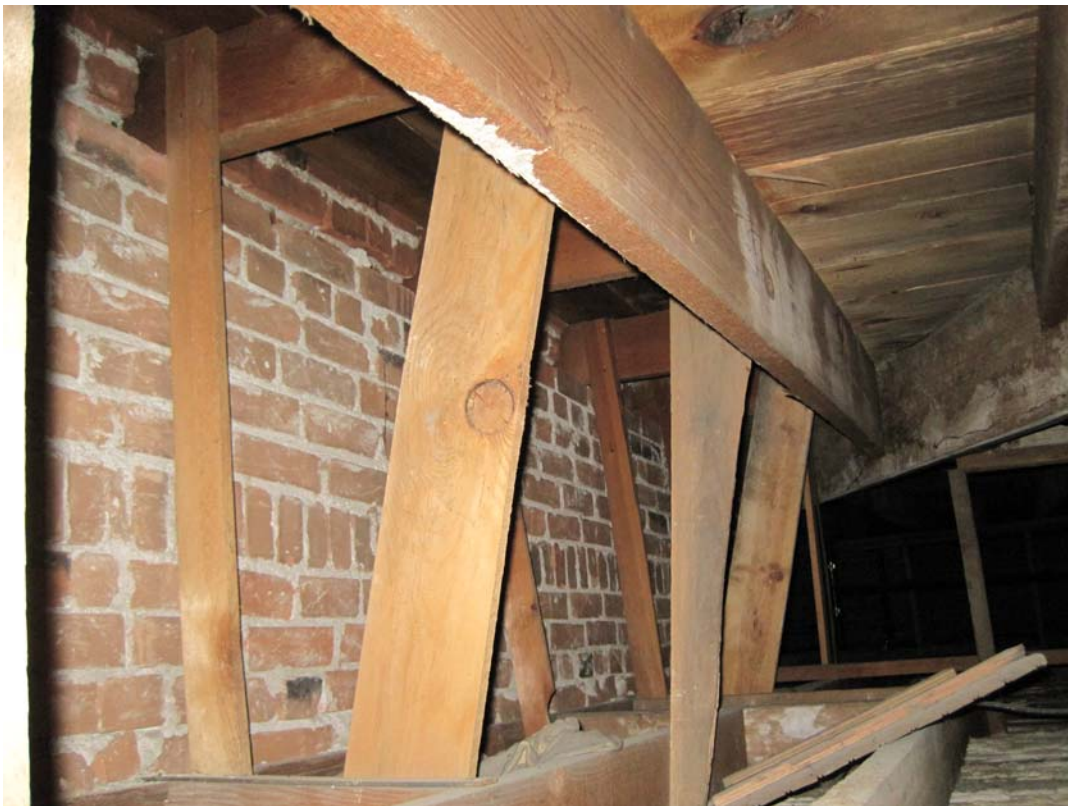
LEL7801 CANTILEVERED CORNICE SUPPORT FRAMING FOR NORTH LIGHT WELL CORNICE ON SOUTH ROOF
