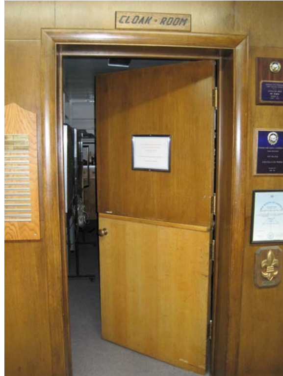
LEL7870 REDESIGNED "DUTCH" DOOR AT FIRST FLOOR CLOAK ROOM
