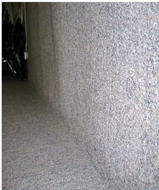
LEL7528 BULGING CARPET WAINSCOT INDICATING SPALLING BEHIND
