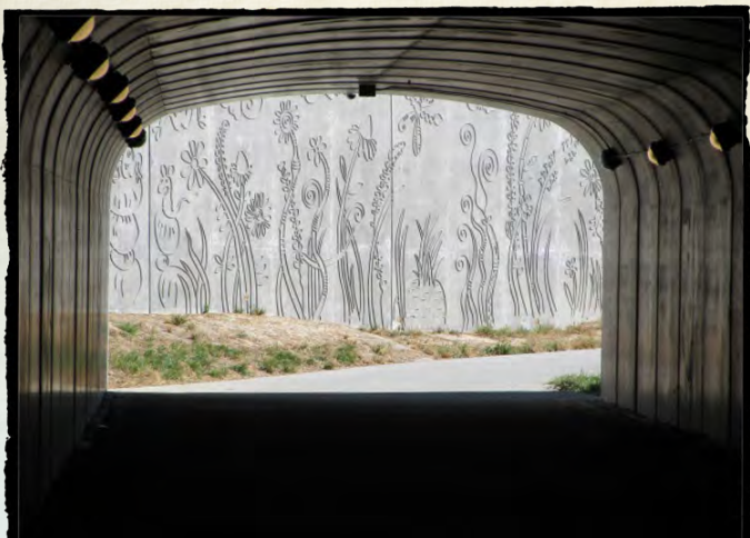
North Highway 287 Recreation Trail Underpass with Concrete Artwork
